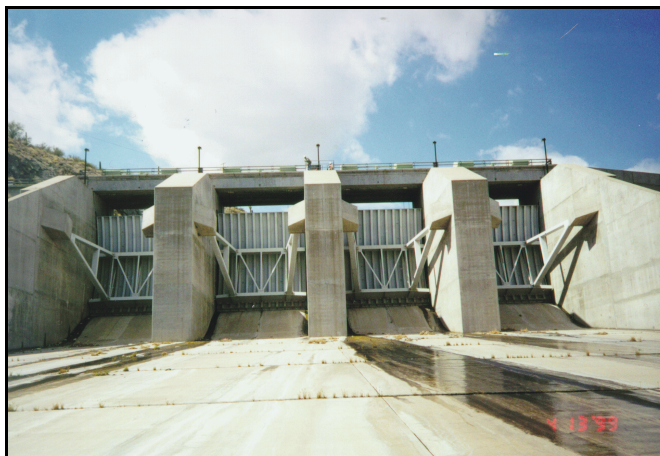
Figure 1.—Downstream side of the auxiliary spillway radial gates (Stewart Mountain Dam).
