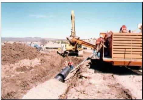
Figure 5.—Open trench without box, gravel uncontrolled.
