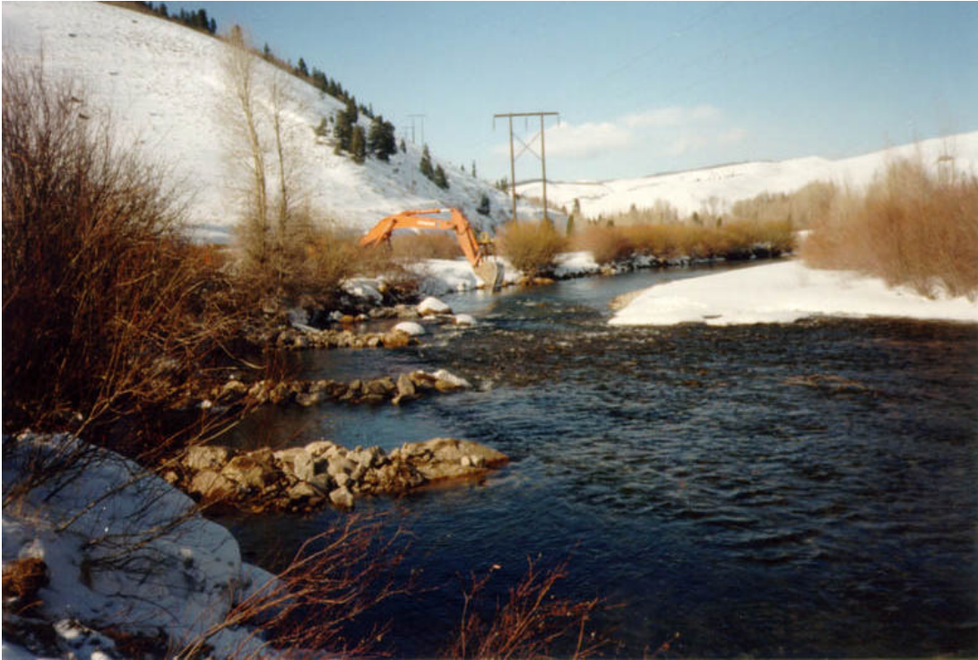
Figure 6.—View looking downstream while weirs are under construction.
