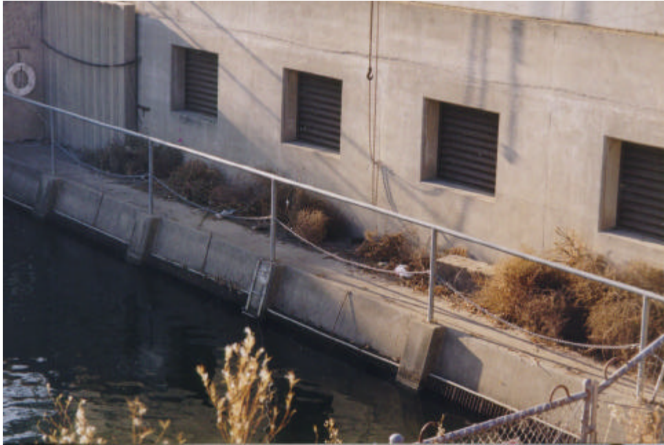
Photograph 1.—Typical inlet area to each pumping plant.
