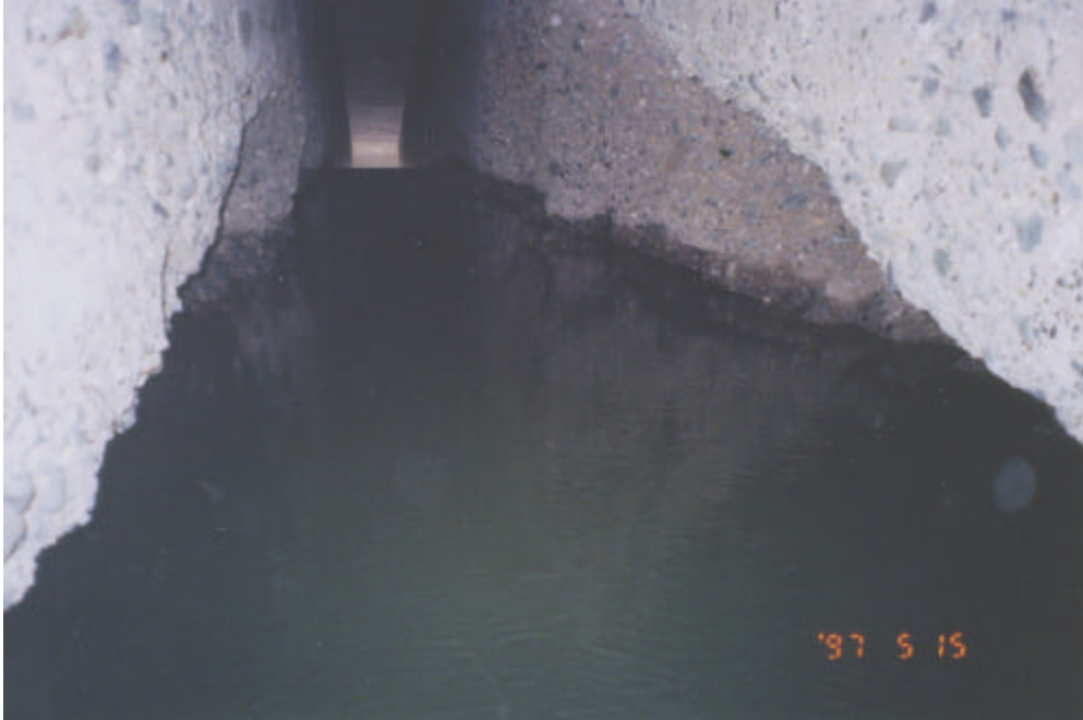
Photograph 1.—Inside river outlet No. 3 looking downstream.
