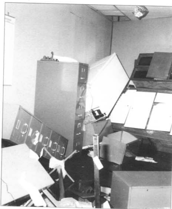
Heavy file cabinets, refrigerator, and other office furniture and equipment "rearranged" in an office area damaged by water.
