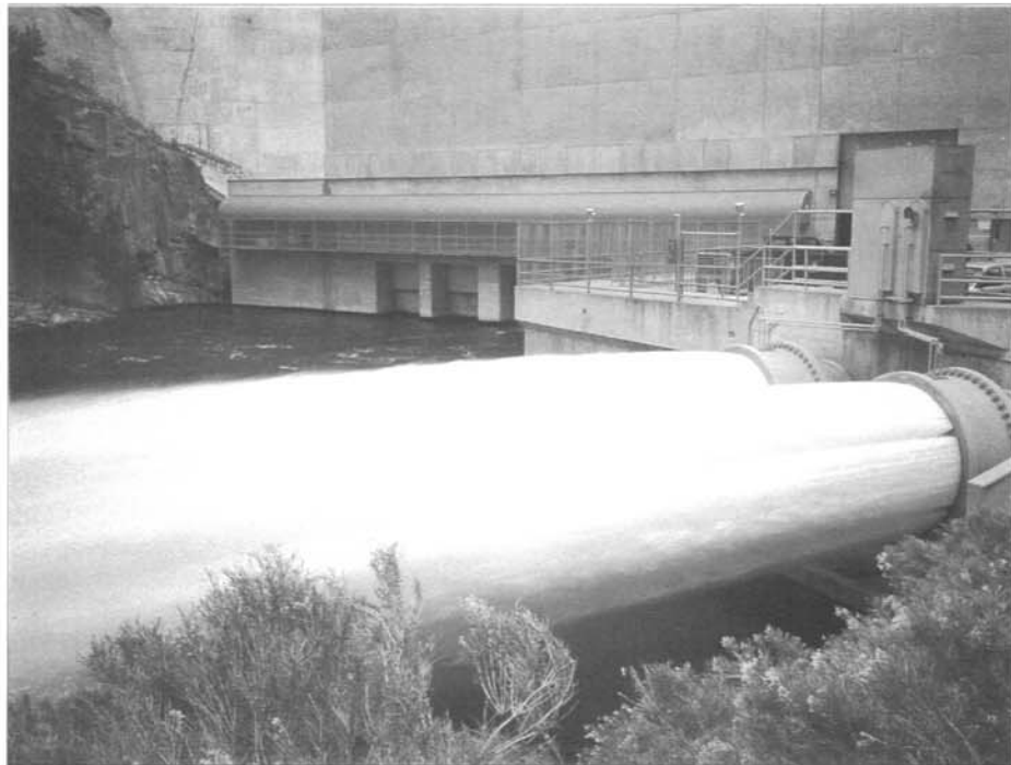
Water gushes at 4,000 cubic feet per second from two 72-inch steel outlet tubes running through Flaming Gorge Dam. Photograph by Tom Ryan (regional office in Salt Lake City, Utah).
