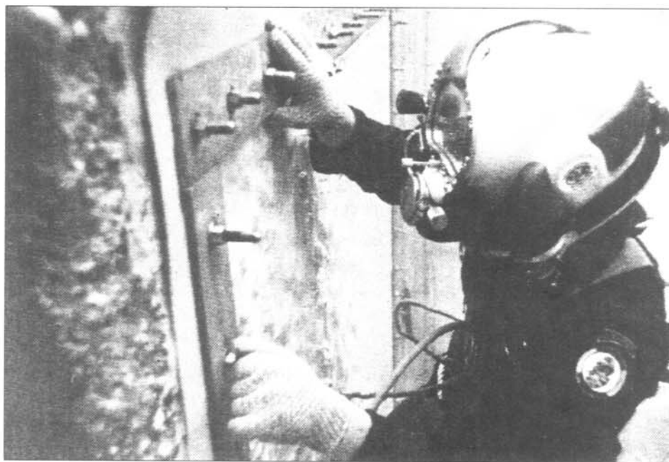
Figure 8.—Membrane tightly conformed to the substrate.
