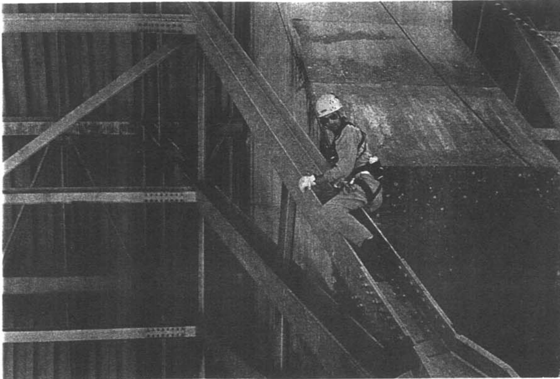
Examination of radial gate at Folsom Dam.
