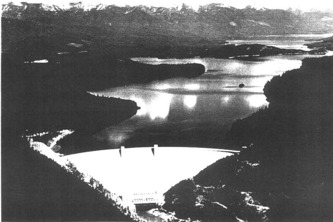
Hungry Horse Dam—564-foot-high thin arch dam located on the South Fork of the Flathead River system.
