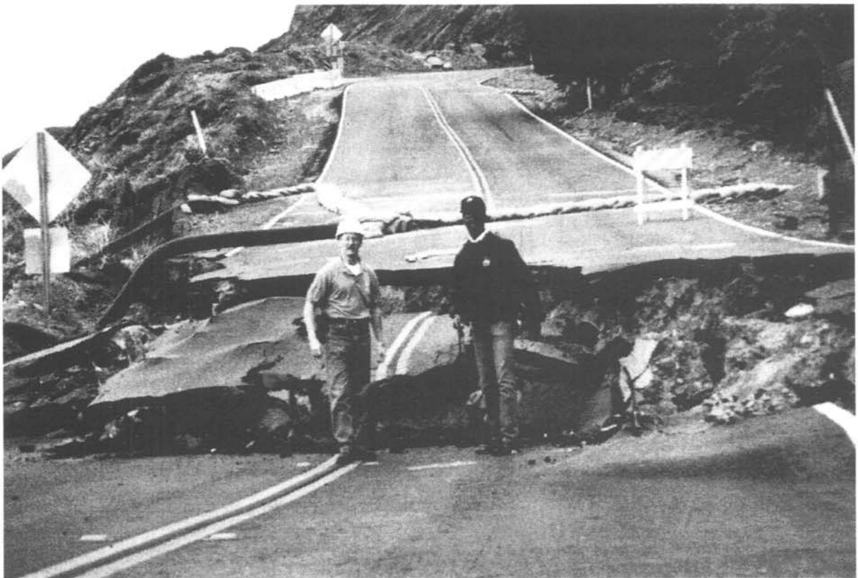
Bureau of Reclamation and California Office of Emergency Services Damage Survey Report Inspectors at the Devils Slide caused by flooding in 1995 in northern California.
