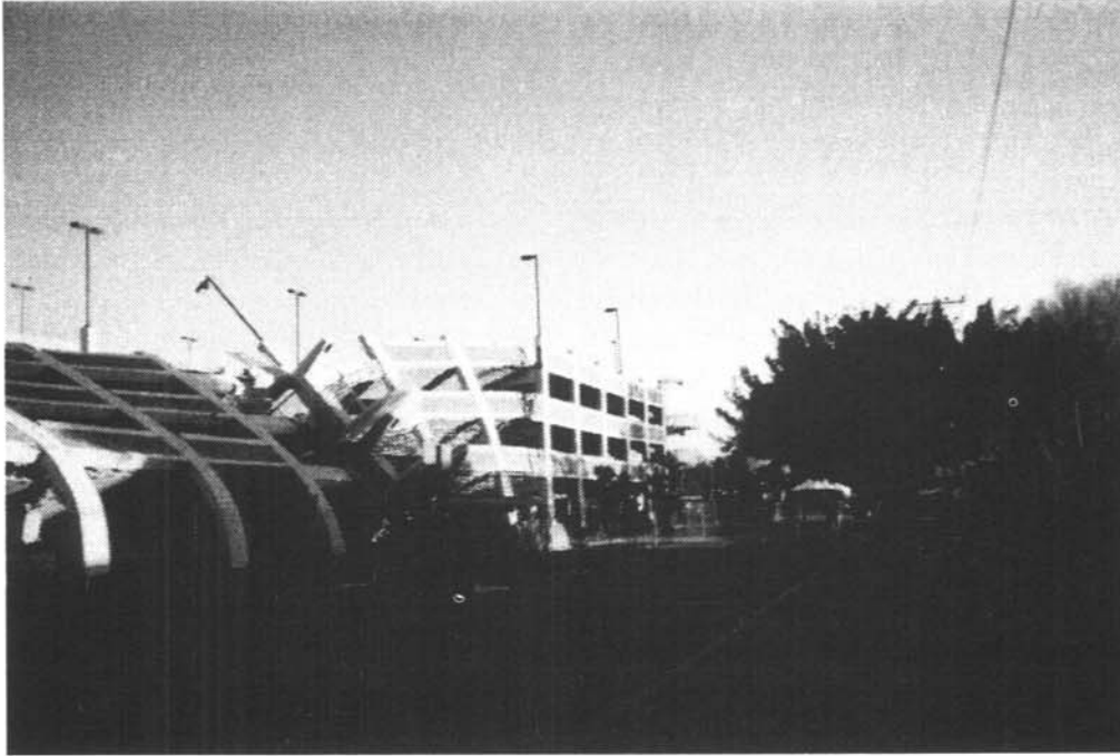
Damage to Cal-State Northridge Campus from the January 1994 Northridge earthquake in Los Angeles, California.
