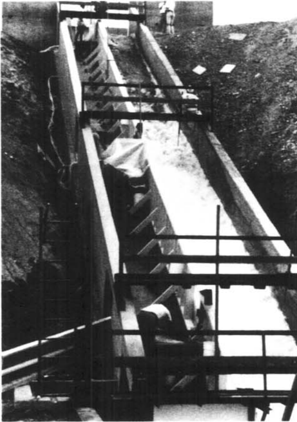
Figure 9.—Large-scale, 15-meter- (50-foot-) high dam overtopping test facility, q = 3 cubic meters/second/meter (32 cubic feet/second/foot).
