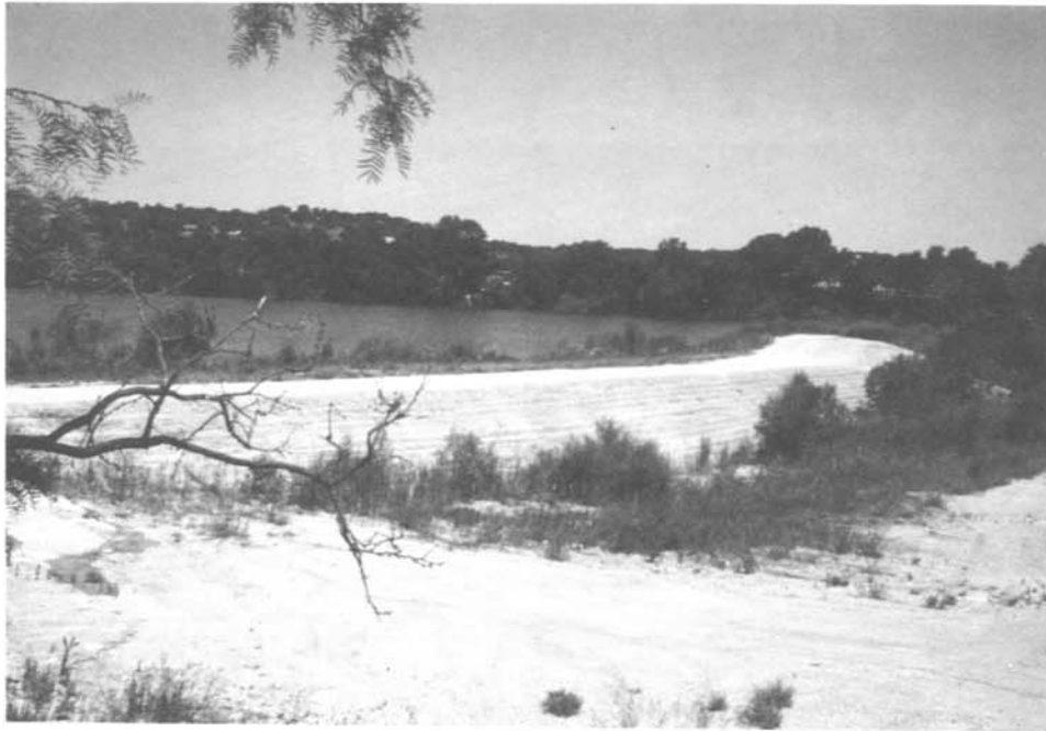
Figure 18.—Brownwood Country Club Dam.
