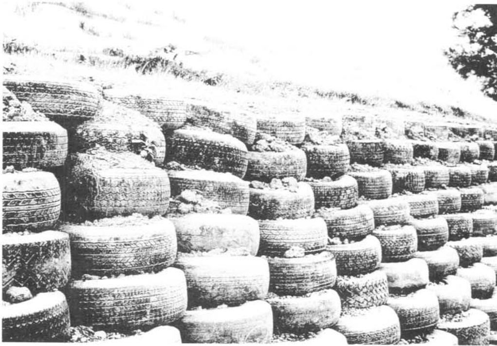
Figure 3. – Used automobile tires being recycled as slope revetment.
