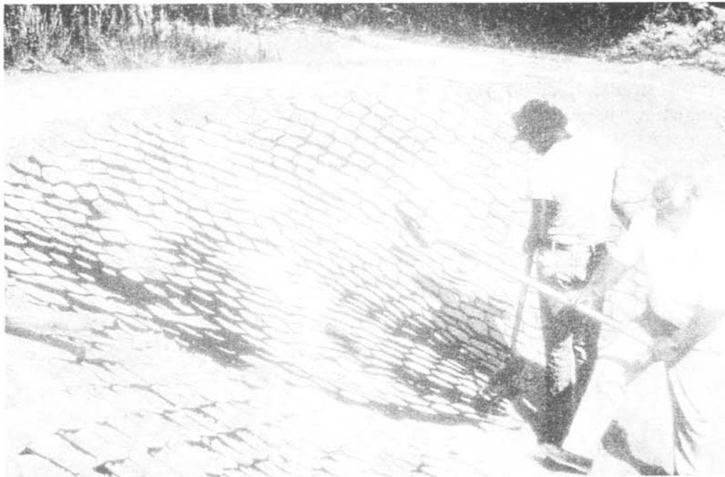
Figure 2. – Geocells being installed on slope to prevent erosion and foster vegetation establishment.
