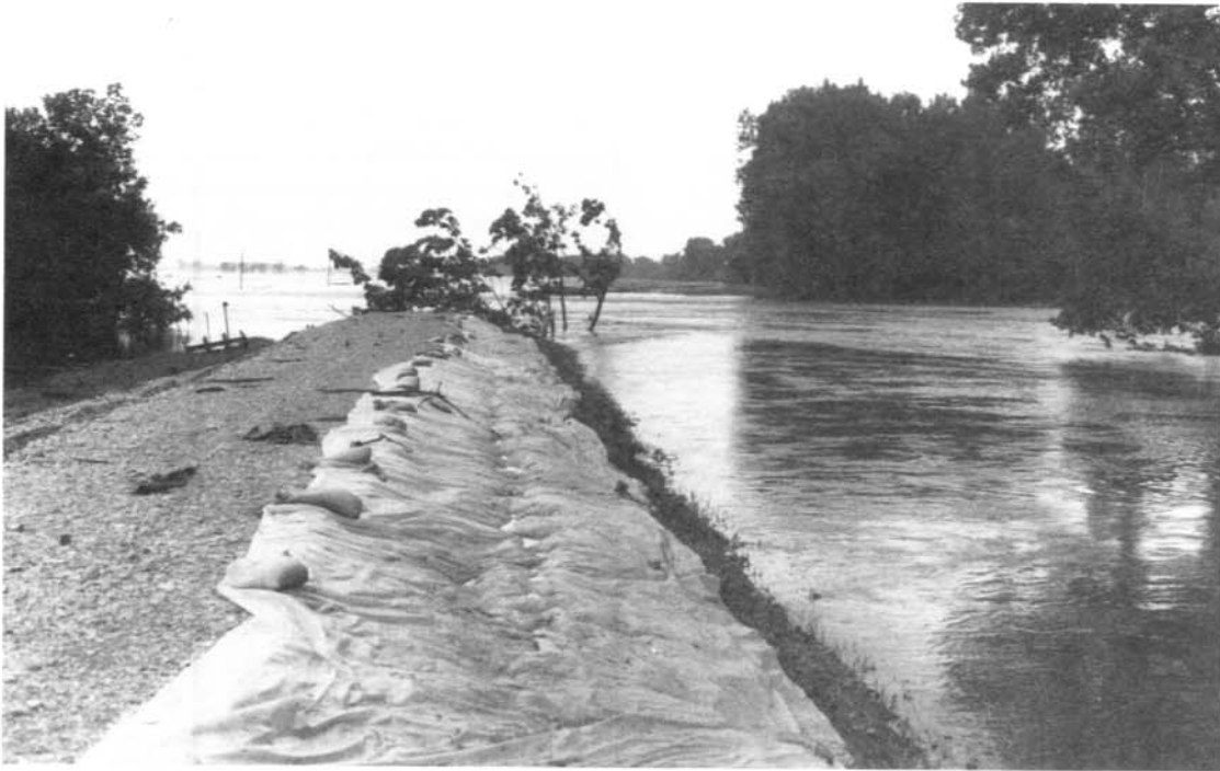
Overtopping of levee, Columbia, IL (photo courtesy of George Sills, Vicksburg District).
