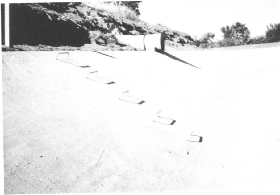
Photo 7.-Finished lining with escape ladder shown.
