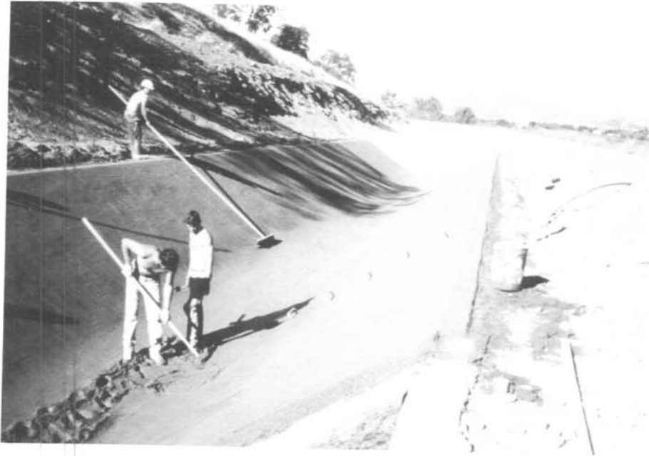
Photo 5.-Finishing surface of shotcrete.
