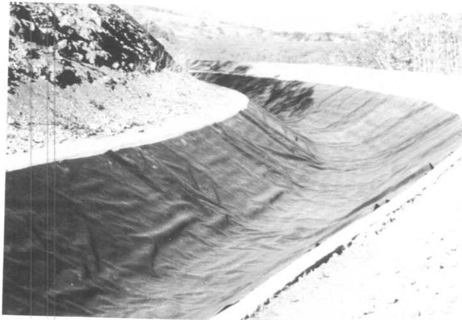
Photo 2.-HDPE liner seamed and in place.
