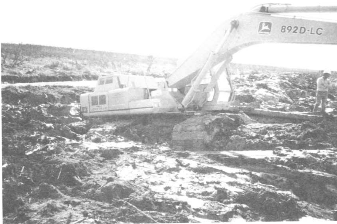
Photo 4. – Conventional excavator mired in Elephant Butte delta after slipping off mats.
