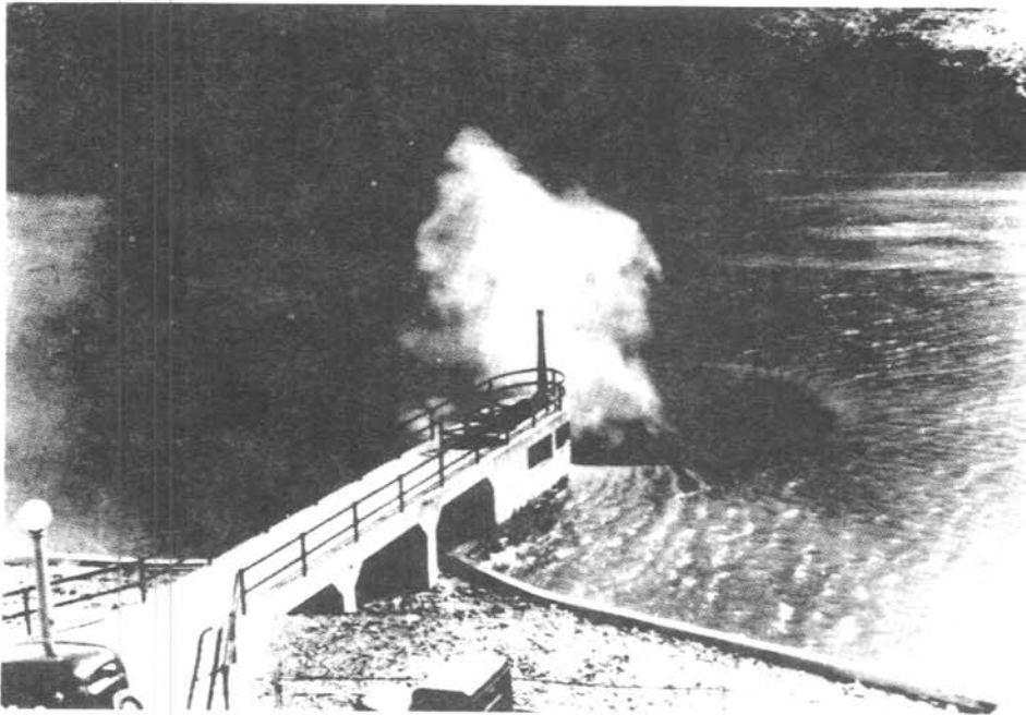
Figure 2. — Observed air blowback in morning-glory spillway at Owyhee Dam, Oregon.
