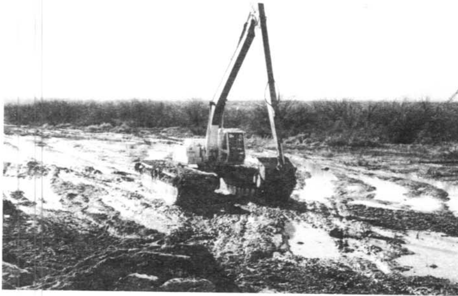
Photo 1. - Amphibious excavator being used in Elephant Butte Reservoir delta. 11/28/90
