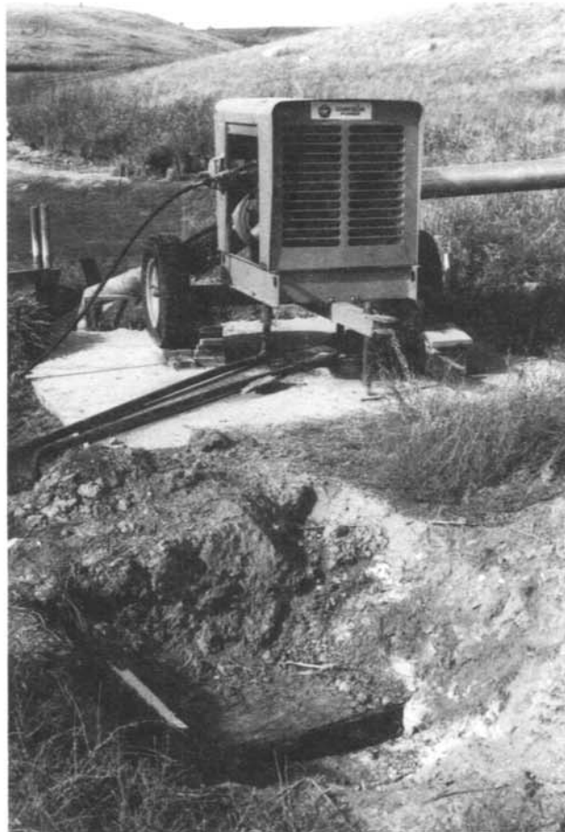
Sound-deadening box partially uncovered.
