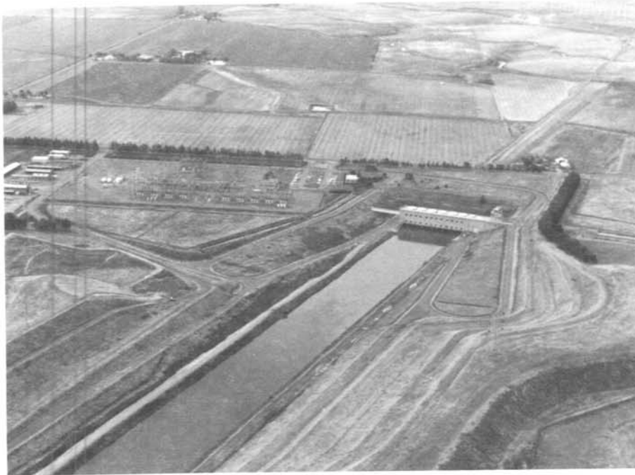
Photo 1. - Aerial view of Tracy Pumping Plant Complex looking upstream showing office area, switchyard, and pumping plant. Water is lifted by this plant 197 feet into the Delta-Mendota Canal. The plant has six pumps, each powered by 22,500-hp electric motors and capable of pumping at the rate of 767 ft 3 /s. Power to run the plant is supplied by Central Valley Project powerplants. 4/12/89
