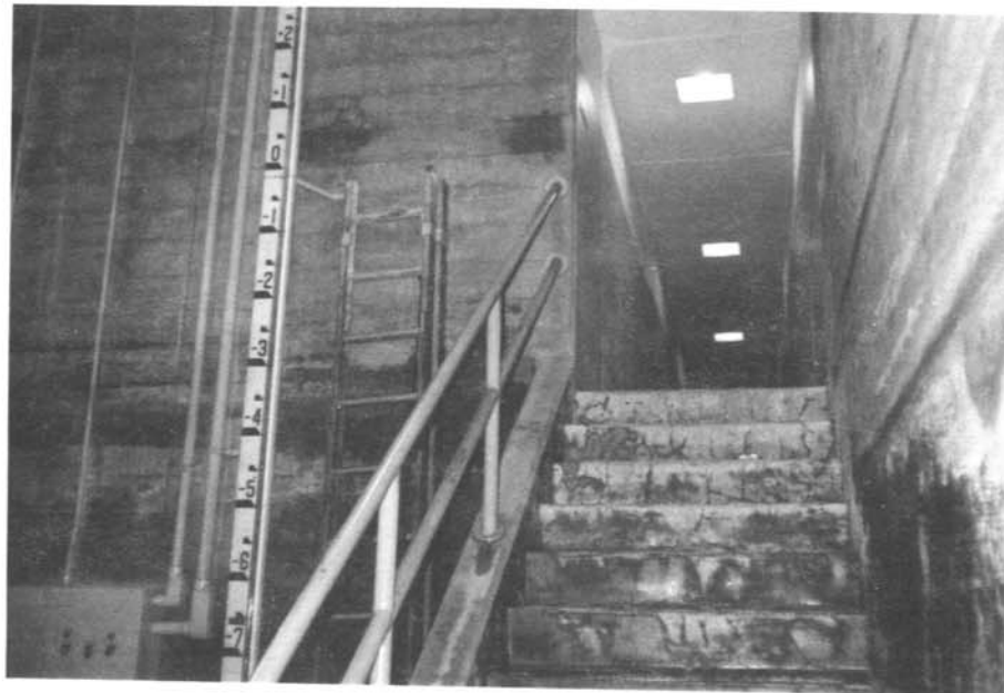
Photo 8. - Unit 5—Water level reached to just above -2 on staff gauge at its highest point. The water level was about 18 inches above the top step in this view. 1/18/91
