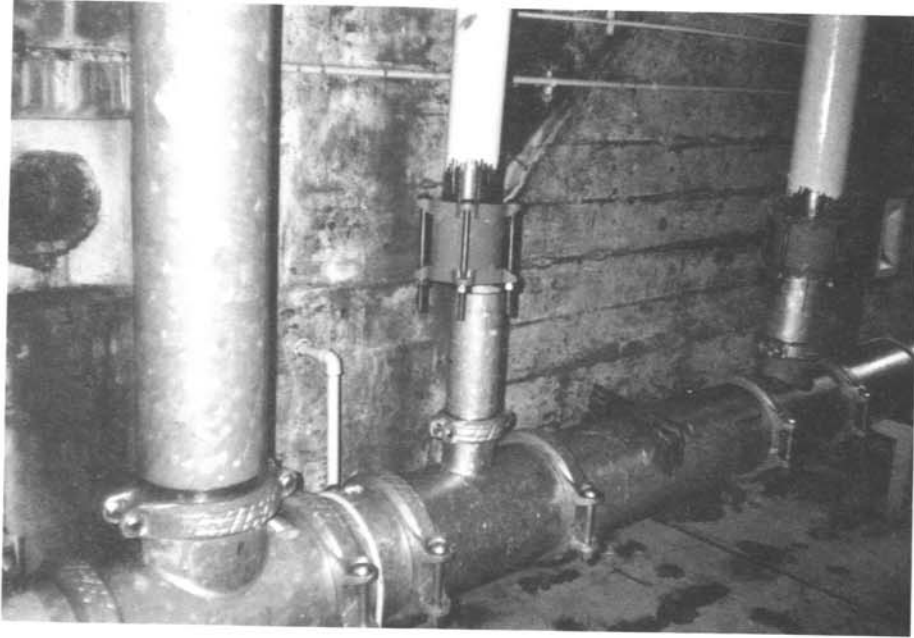
Photo 3. - Unit 5—4-inch sleeve coupling, one of two that came apart. Coupling is typical of all. Note also the unrestrained 6-inch sleeve coupling at the right of the photo. 1/18/91
