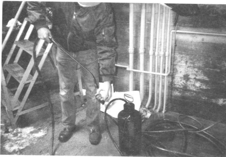
Photo 12. - Unit 4—Cleaning electrical component with water. 1/18/91
