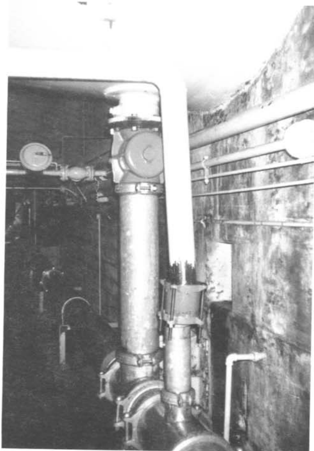
Photo 3. - Unit 5—4-inch sleeve coupling, one of two that came apart. Coupling is typical of all. Note also the unrestrained 6-inch sleeve coupling at the right of the photo. 1/18/91
