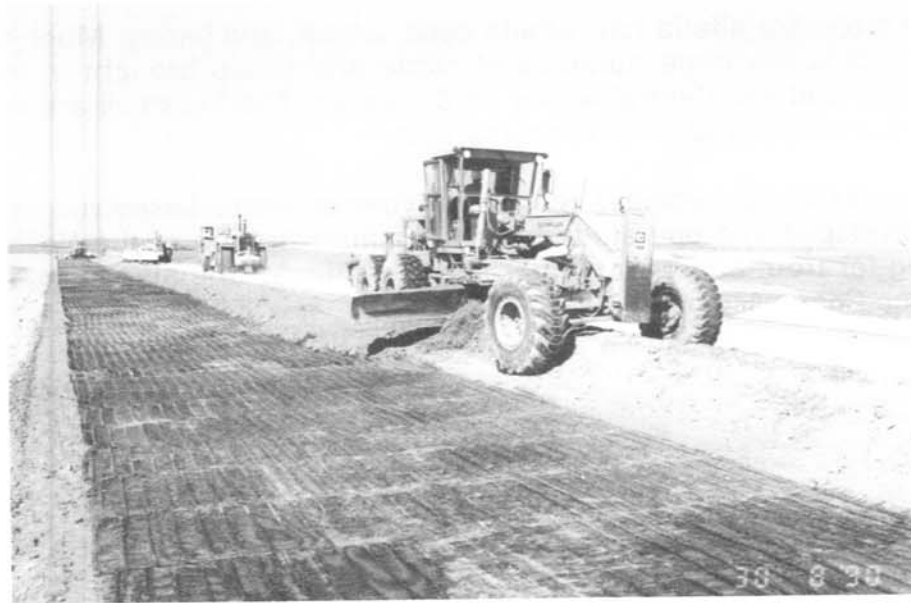
Geogrid placement at Davis Creek Dam.
