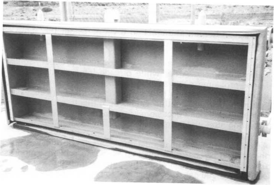
Duct tape over neoprene seals on large bulkhead gate at Stampede Powerplant.
