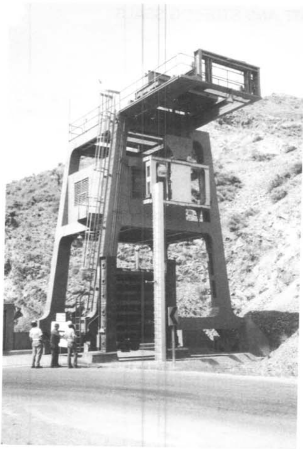
Bulkhead gate stored below gantry crane at Canyon Ferry.
