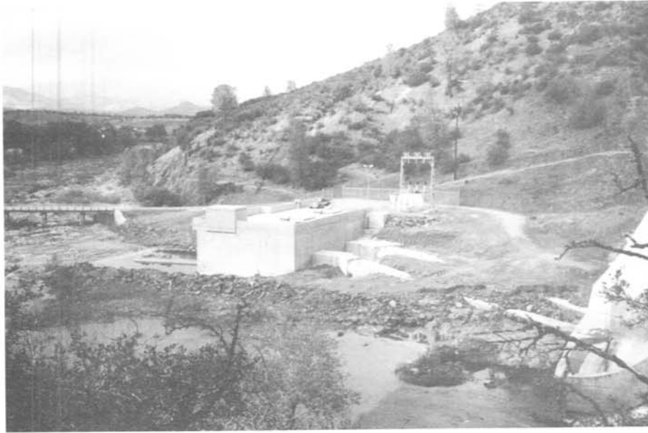
Figure 3. - City of Santa Clara powerplant immediately downstream of Stony Gorge Dam. Photo by Bill Bouley. 10/26/89
