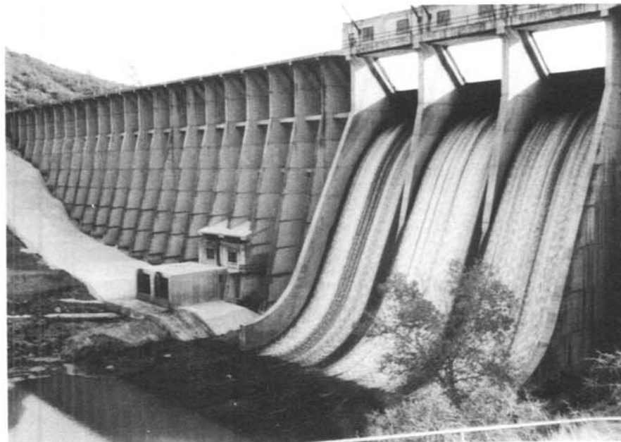
Figure 2. – Downstream view of Stony Gorge Dam showing the overtopping protection at the base of the dam. Photo by Joan Goodwin. 10/26/89
