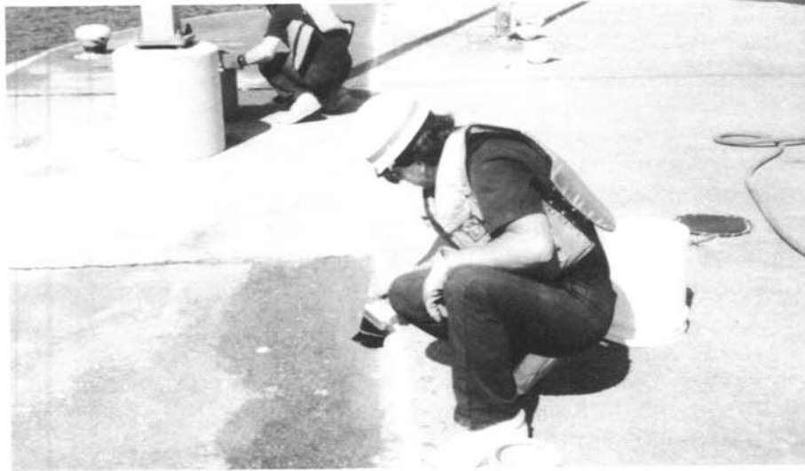
Field testing of a penetrating concrete sealer, Brandon Road Lock and Dam, Rock Island District, Illinois.
