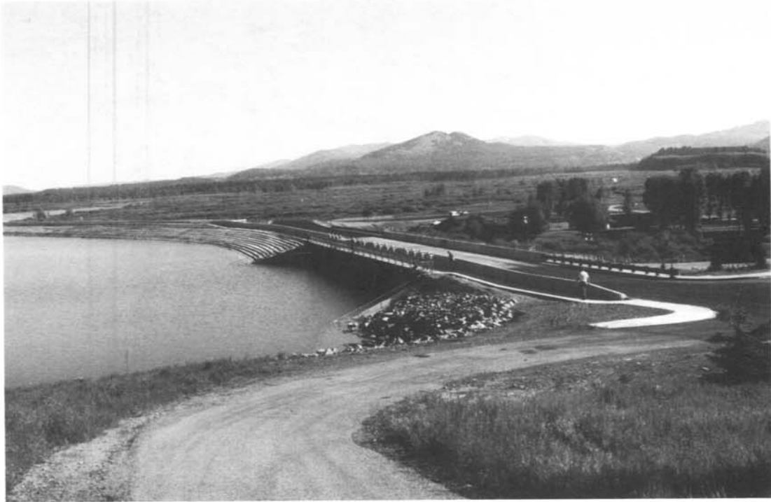
Photo 3. - View of Jackson Lake Dam and Reservoir at water surface elevation 6766.8. — Bureau of Reclamation photo by S. Bareis. 6/27/89
