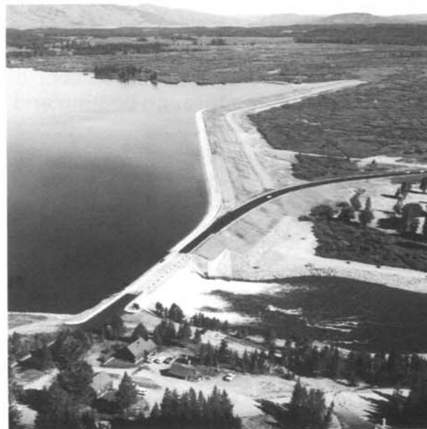
Photo 2. - Aerial view looking north showing general view of Jackson Lake Dam with a full reservoir elevation 6769.0. Releases from the reservoir were 1700 ft 3 /s at time photo was taken. — Bureau of Reclamation photo by Glade Walker. 7/17/89
