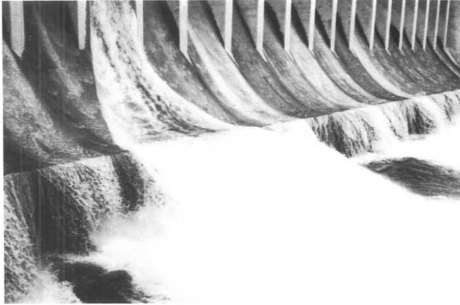
Photo 7. - Jackson Lake Dam spillway radial gate discharge. — Bureau of Reclamation photo by Bill Bouley. 7/27/89
