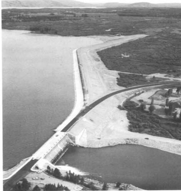
Photo 1. - Aerial view of Jackson Lake Dam looking north from south side of river showing completed dam and progress of reservoir filling. Reservoir is at elevation 6765.4 (maximum elevation is 6769.0). — Bureau of Reclamation photo by G. Walker. 6/20/89
