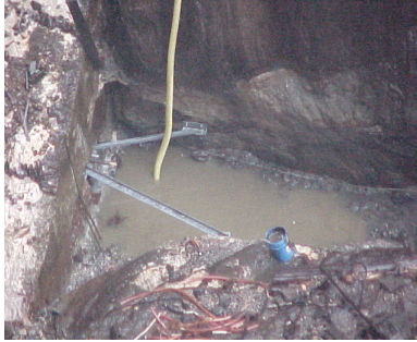
Steel angle bracing of bulkhead.
