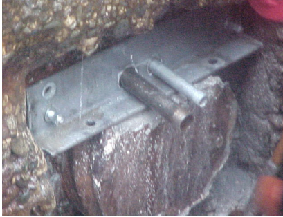
Steel angle bulkhead.
