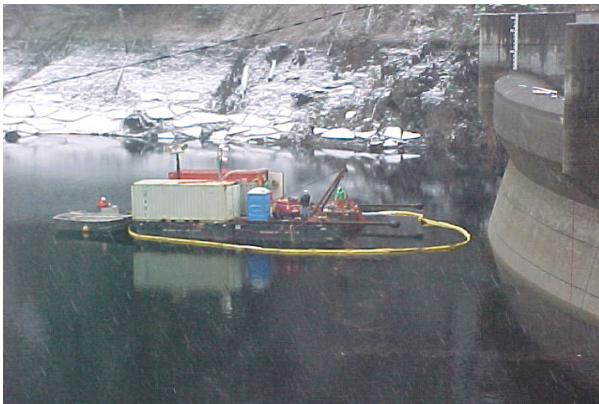
Work barge on station above Conduit 4-165.
