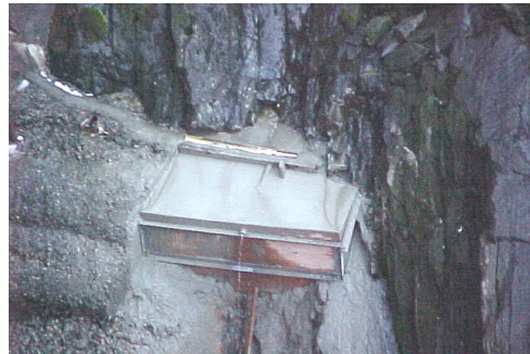
Conduit 3-196 downstream end, new concrete encapsulation.
