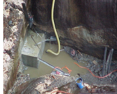
Concrete cap on Conduit 4-165 downstream end.
