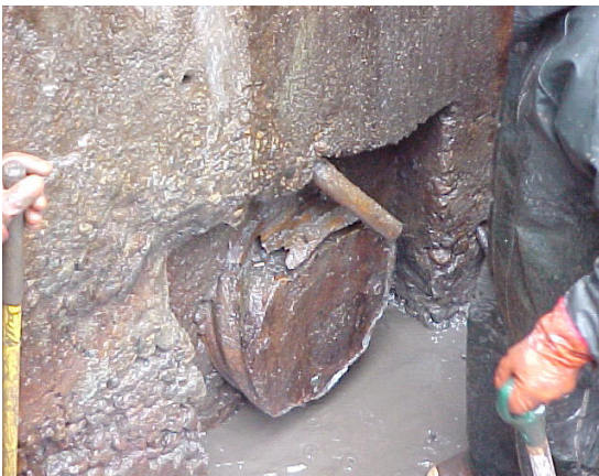
Conduit 4-165 damaged downstream end.
