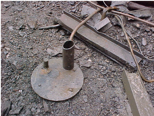
Original end cap and waler system.
