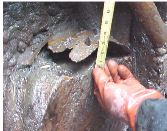
Conduit 4-165 damaged downstream end.
