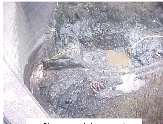
Plunge pool dewatered
