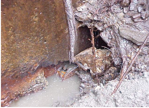
4-165 downstream end revealed.
