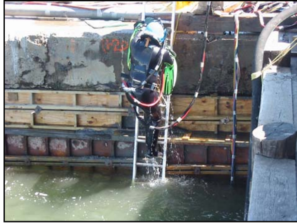
Underwater construction inspections act as countermeasures against contractor claims.
