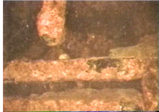
Conduit 4-165 upstream end, view from mid-height right side of block-out.
