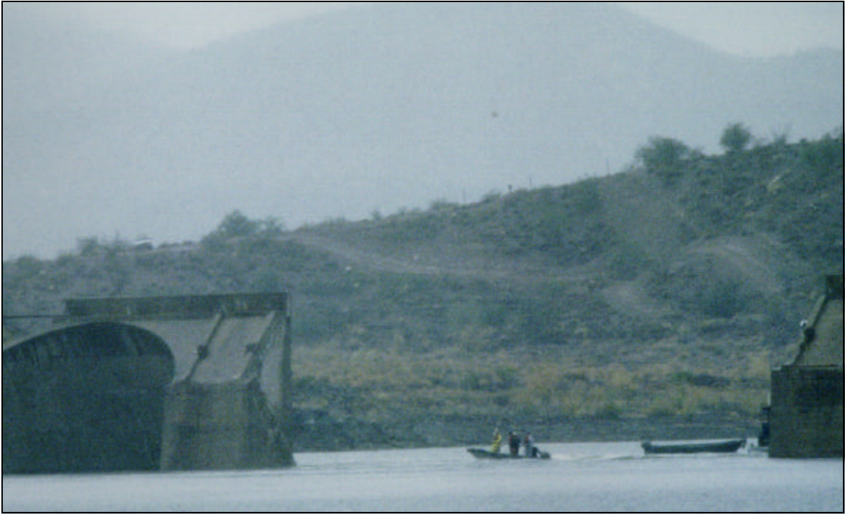
A breach is created in historic Waddell Dam.
