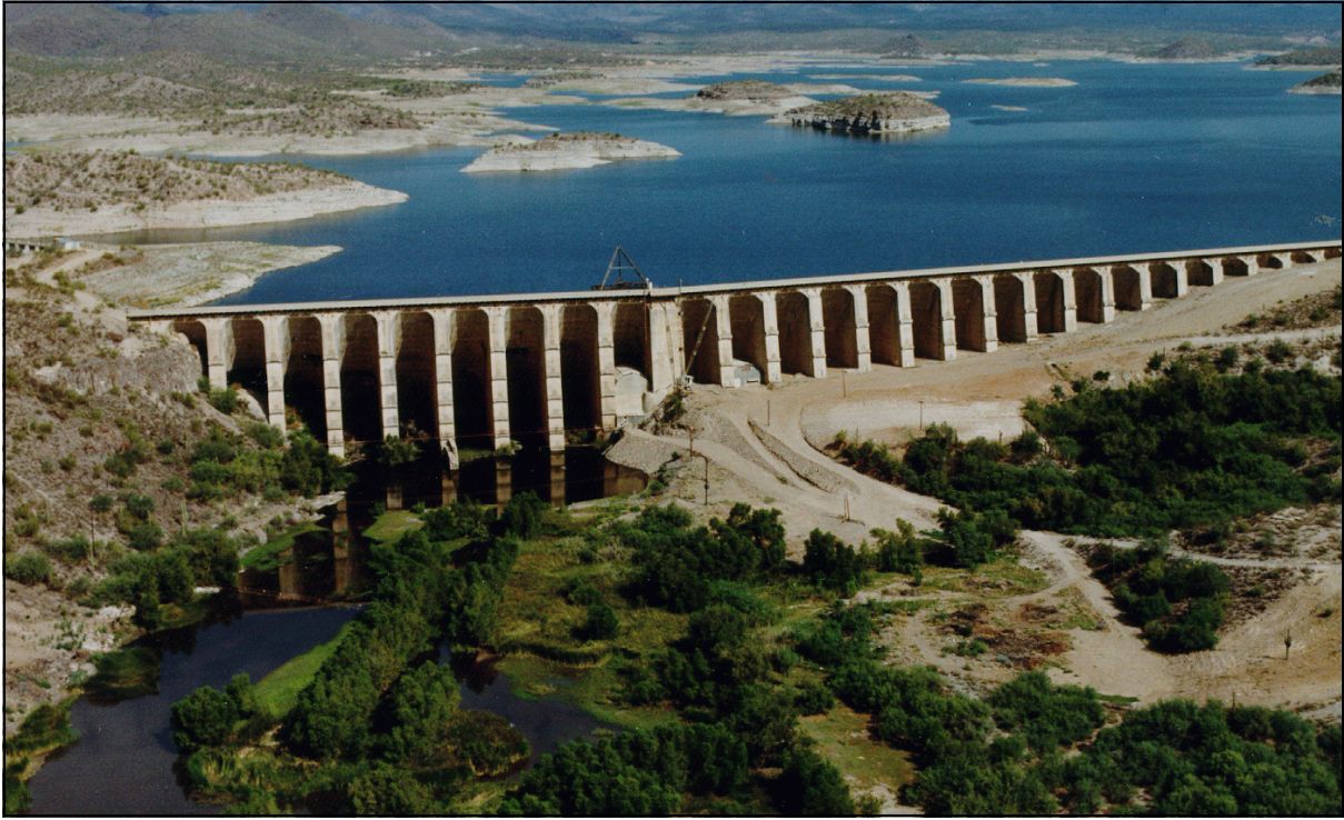
Historic Waddell Dam, constructed in 1927.
