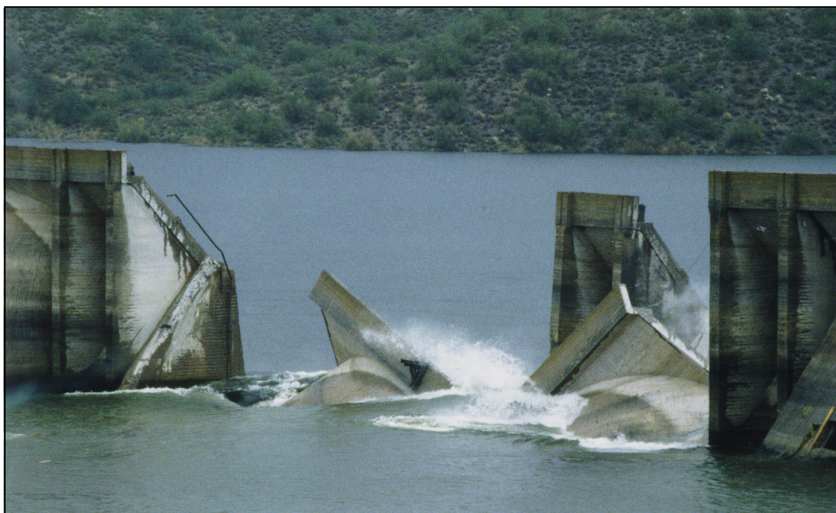
Blocks of concrete from historic Waddell Dam sink into Lake Pleasant.
