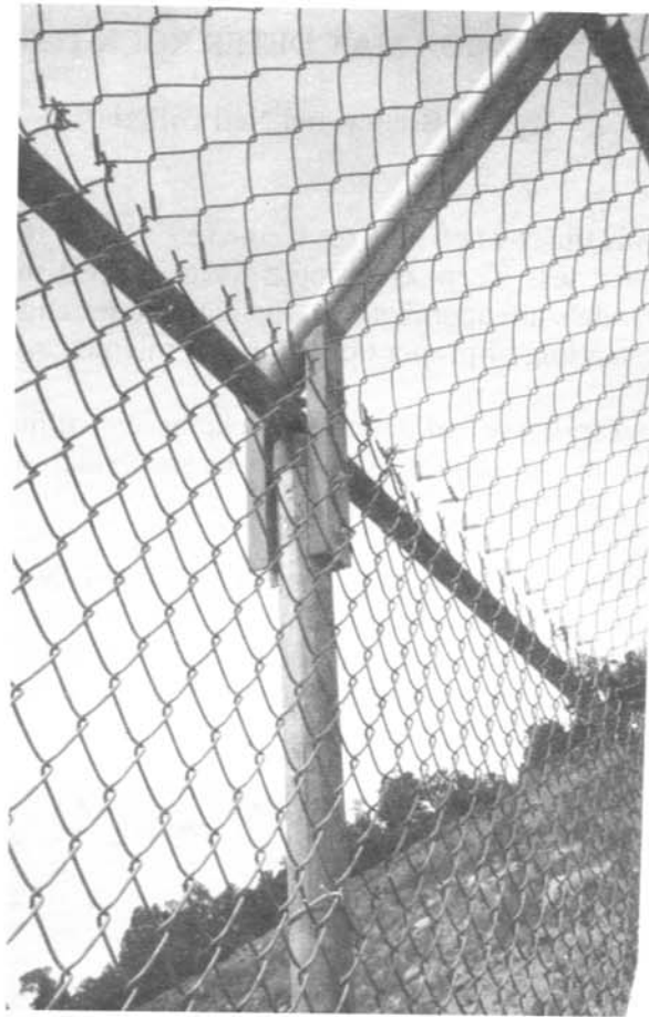
Spillway fence extension connectors.
