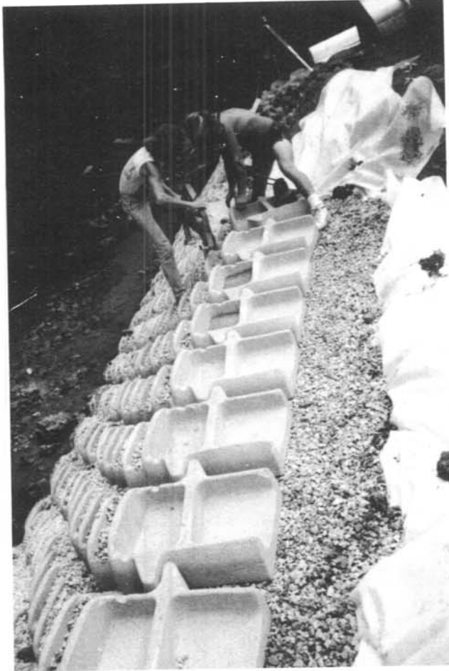
Creek bank stabilization system is built by placing layers of trough shaped modules on the steep slope. Interlocking wings tie units together, as shown in detail at left. Later a scour protection system was placed at the toe.
