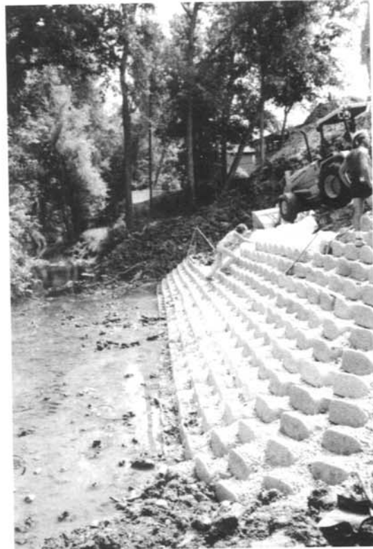
Creek bank stabilization system is built by placing layers of trough shaped modules on the steep slope. Interlocking wings tie units together, as shown in detail at left. Later a scour protection system was placed at the toe.
