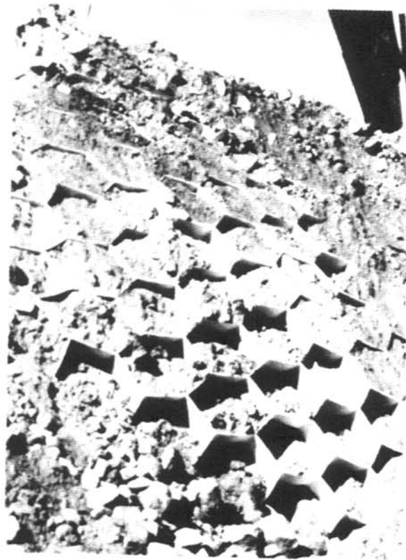
The honeycombs of the Armater were filled with a mixture of rock fine, consisting of baseball- to football-size rocks, and soil to keep the banks stable.
