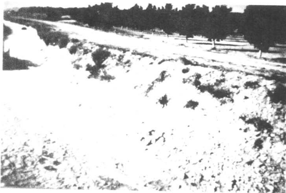
The Elephant Butte irrigation system consists almost entirely of earthen canals, laterals, and ditches.
