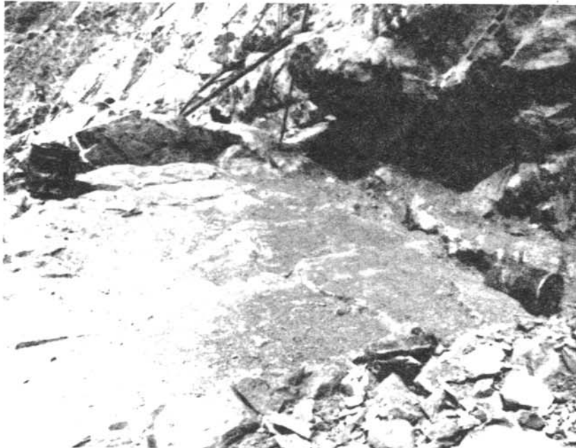
Figure 3. - Overhangs treated with pneumatically applied concrete for foundation shaping.
