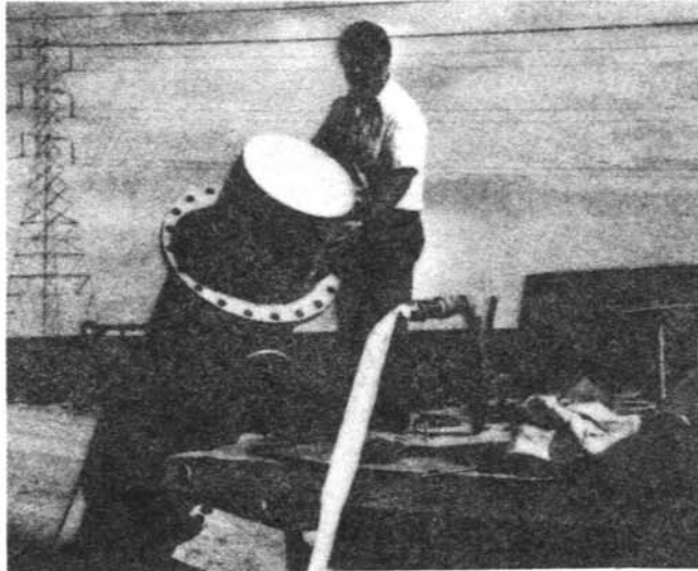
Introducing the "pig" into the irrigation line.
