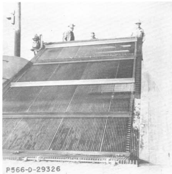
Looking Downstream at Trashrack and Cleaning Device Fig. 188B
