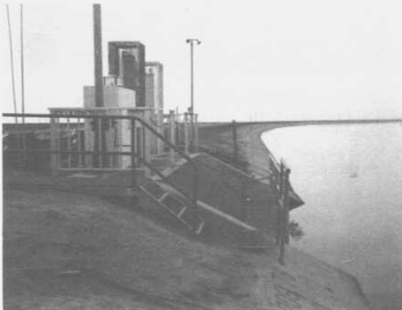
Figure 9.—Typical customer turnout site.
