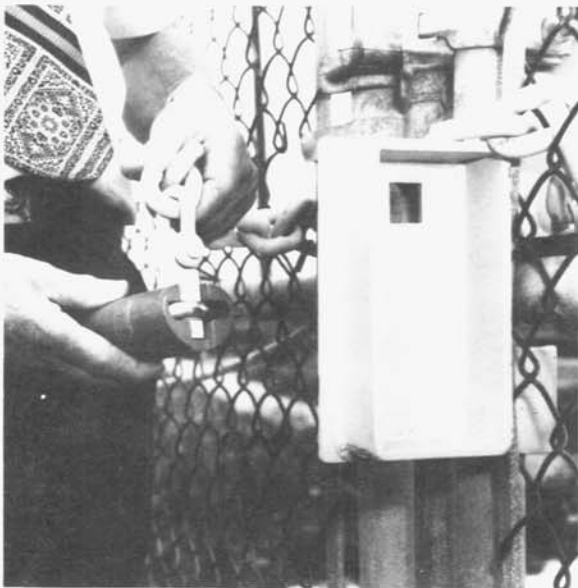
Figure 5.—Slotted-staple hasp box assembly.
