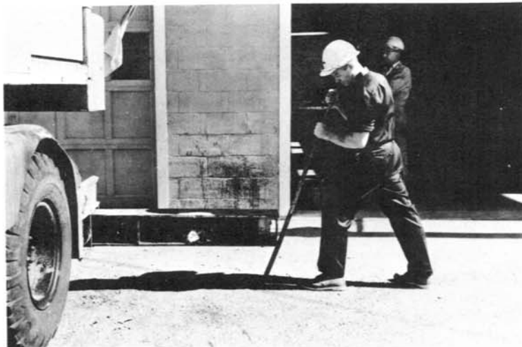
Photograph 2. Photo P245-713-4175 NA
