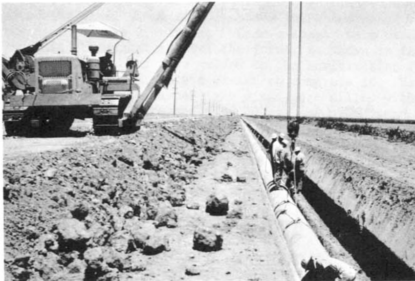
Photograph 1. Photo P805-243-1177 NA
