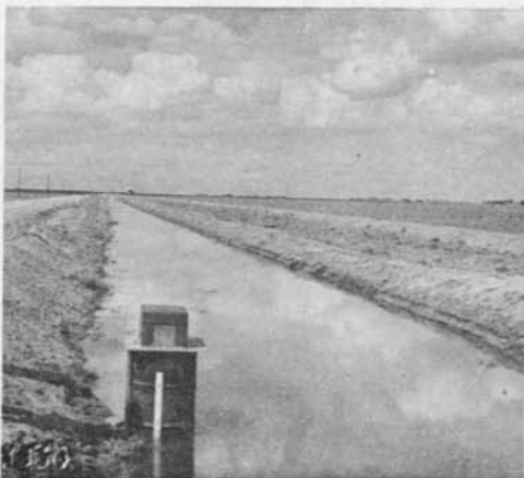
COVER PHOTOGRAPH: This is a view of Recorder Station upstream from Station 581+40, on the Eden Project, Upper Colorado Basin, Wyoming. Photo P153-D-27834
