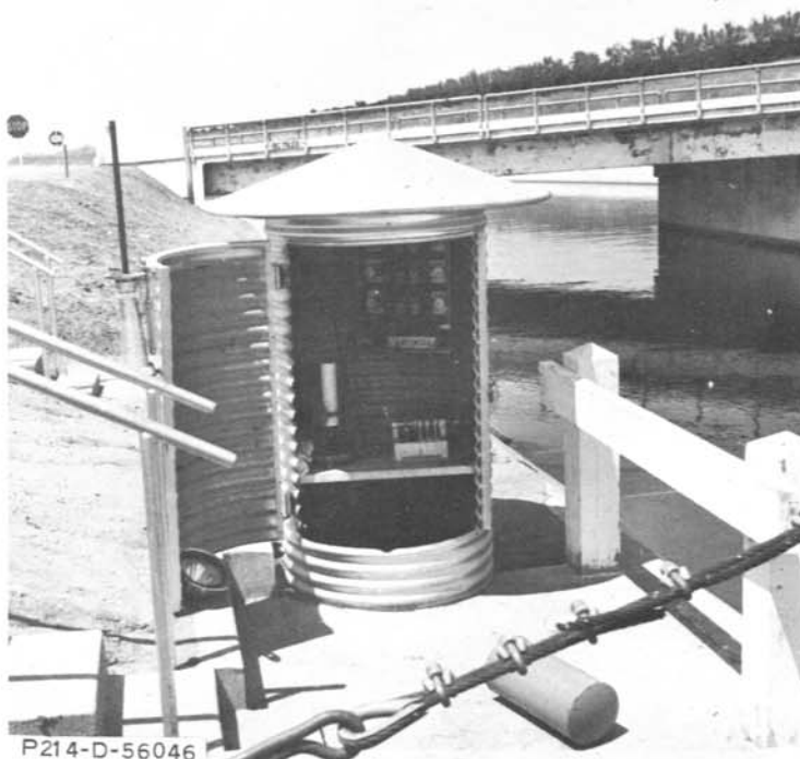
Photograph No. 2-- Recorder Well-- located immediately upstream on right bank. Note auto- matic gate control device.
