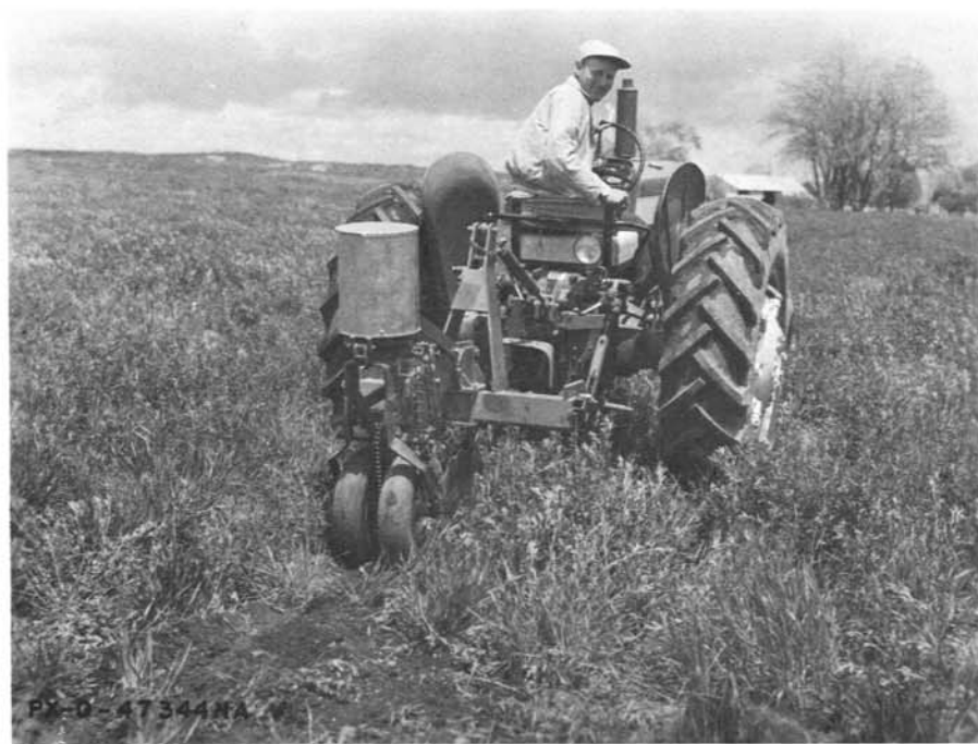
Figure 2--Burrow-builder in operation
