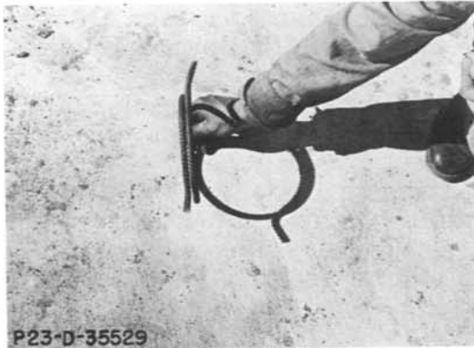
Fig. 1--Re-bar ring made with bender.
