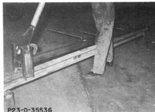
Applying pressure to check gate guide to straighten.
