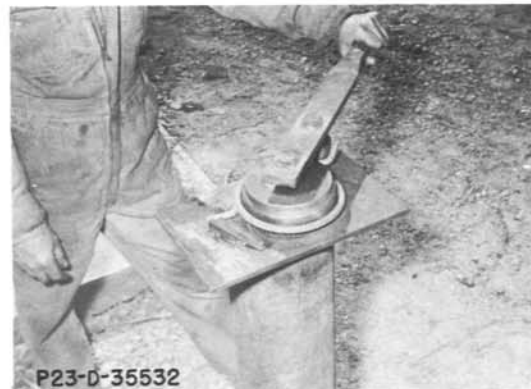
Fig. 4--Bender in final position after bending bar.
