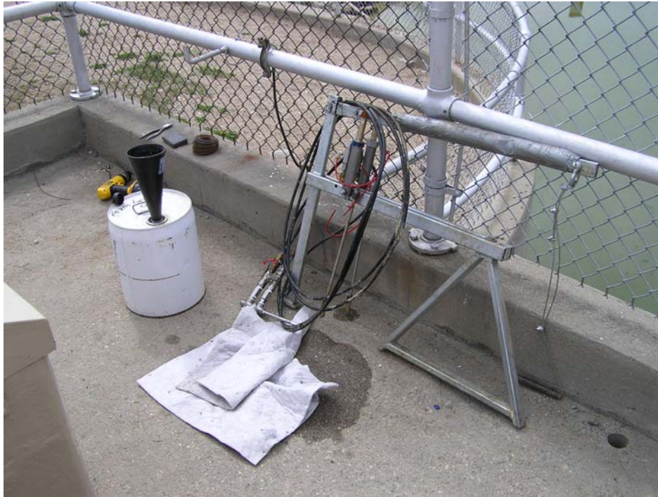
Two-part "Zipper" pump used to inject chemical grout.
