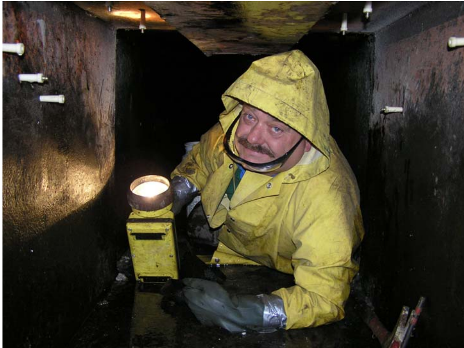
Looking downstream into tight quarters in the outlet works.
