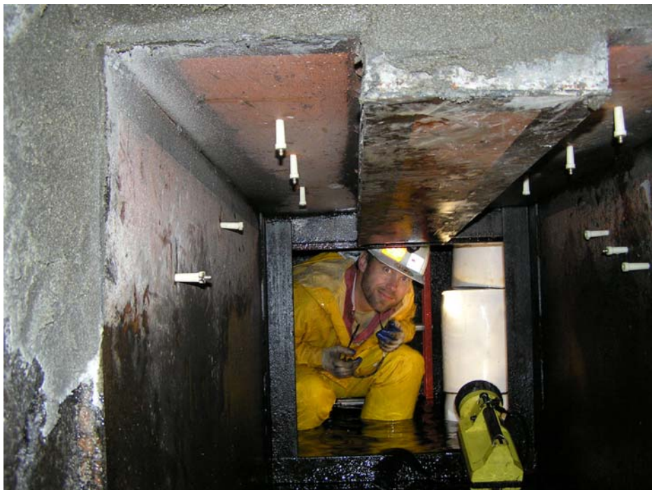
Looking upstream into outlet shaft at pump operator.
