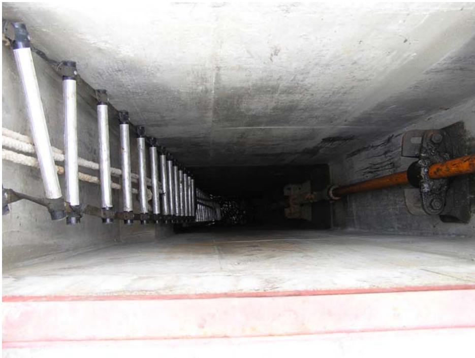
Access to outlet works liner.
