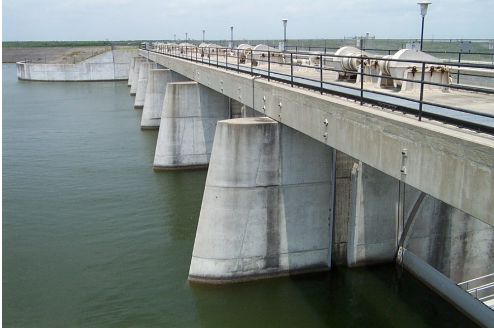
The upstream side of the gated spillway at Choke Canyon Dam.
