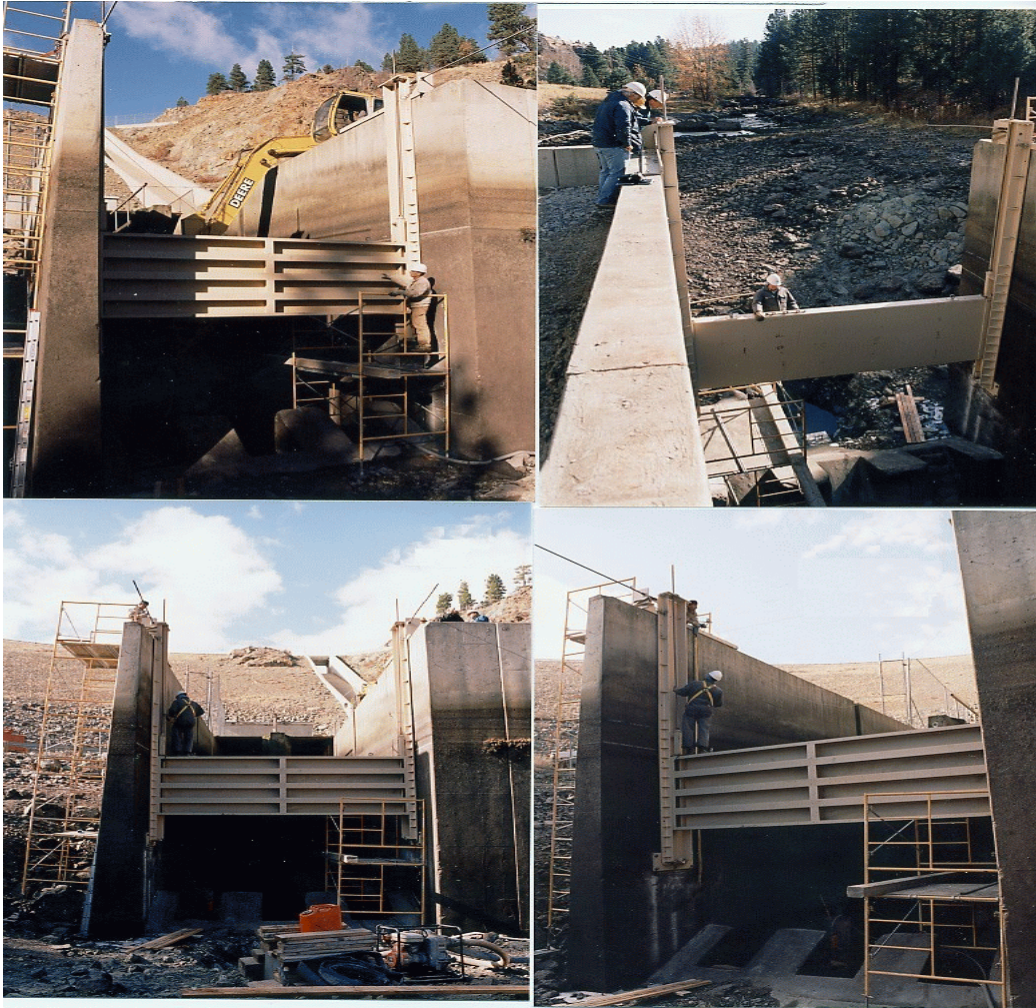
Figure 13.—Prototype flow deflector installation at Mason Dam in October 2002.
