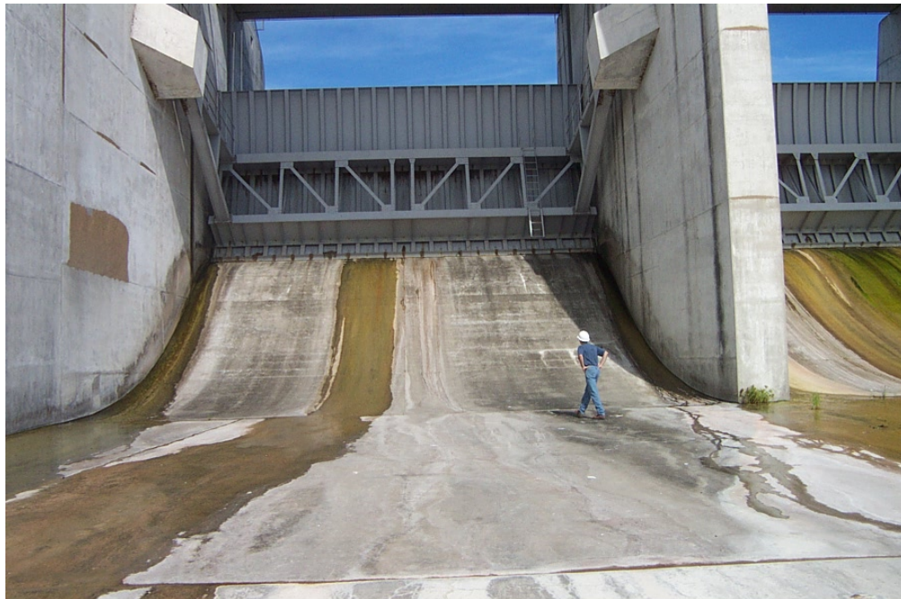
The downstream side of the spillway radial gates at Choke Canyon Dam.
