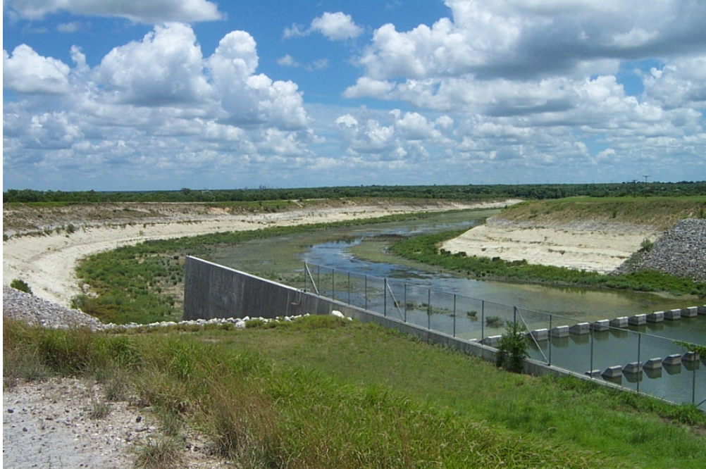
The river channel downstream of the Choke Canyon Dam spillway.
