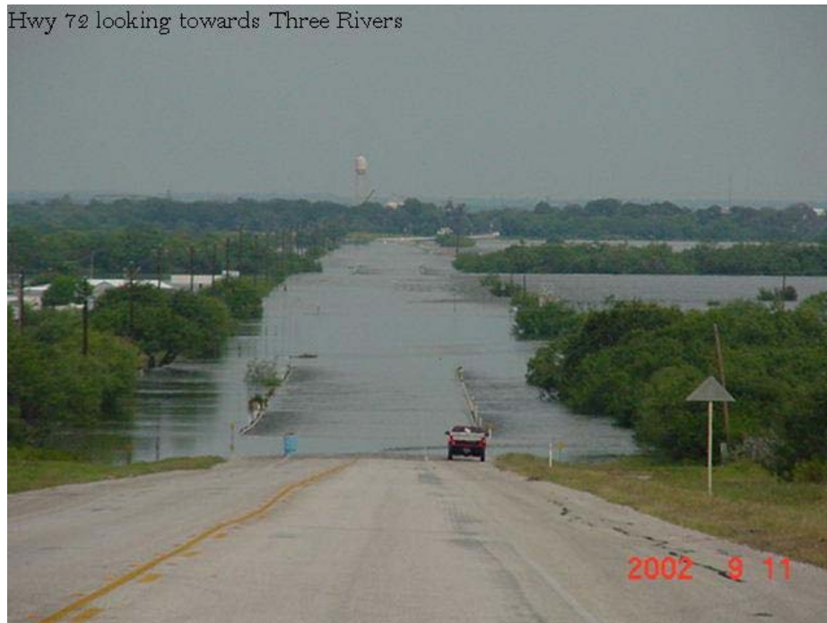
Downstream of Choke Canyon Dam during surcharge operations at State Highway 72 looking (east) towards the city of Three Rivers, Texas, September 2002. Normally, this section of the highway is 1 to 2 miles from the Frio and Atascosa Rivers.
