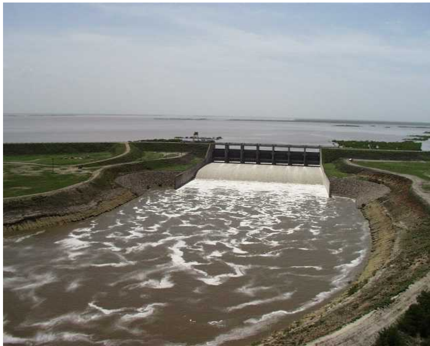
Choke Canyon Dam surcharge releases being made during a July 2002 event.
