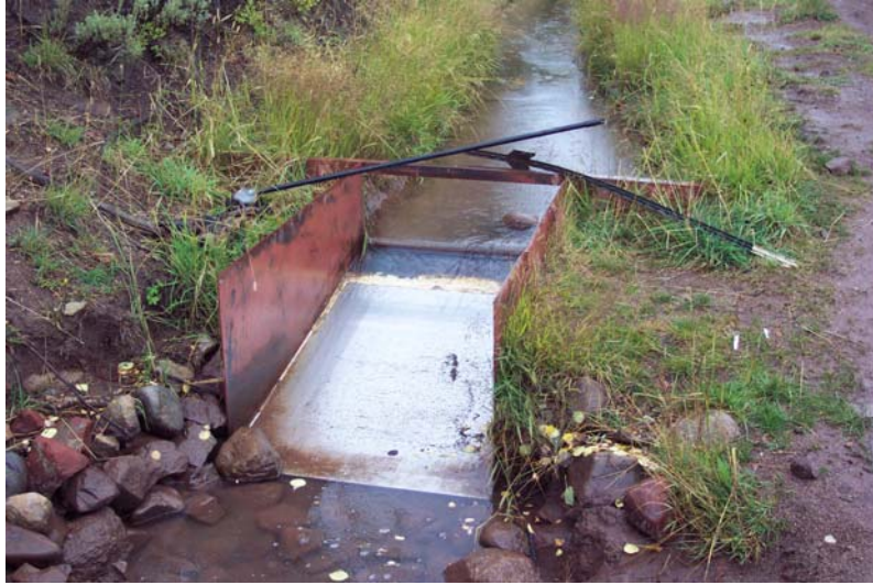
Figure 11.—A small Coanda-effect screen provides water to a sprinkler irrigation system near Carbondale, Colorado.
