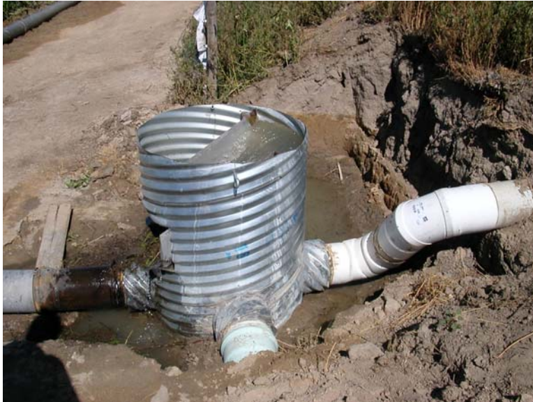
Figure 3.—Coanda-effect screen structure built with corrugated metal pipe. Raw water enters from the right. Clean water is discharged through the center and left-hand pipes, while debris exits onto the ground through the slot in the left side of the structure.
