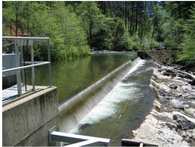
Figure 9.—Montgomery Creek intake.
