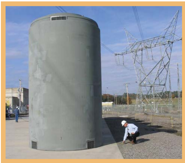
Scott Atwater, Region IV DNMS inspector, checking dry fuel storage casks at Arkansas Nuclear One in Russellville, AK.
