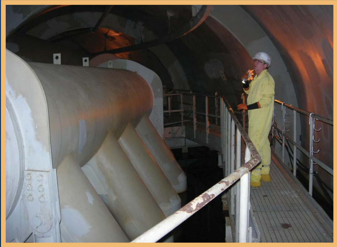
The Monticello Nuclear Power Plant is located in Monticello, MN, 30 miles northwest of Minneapolis, MN
