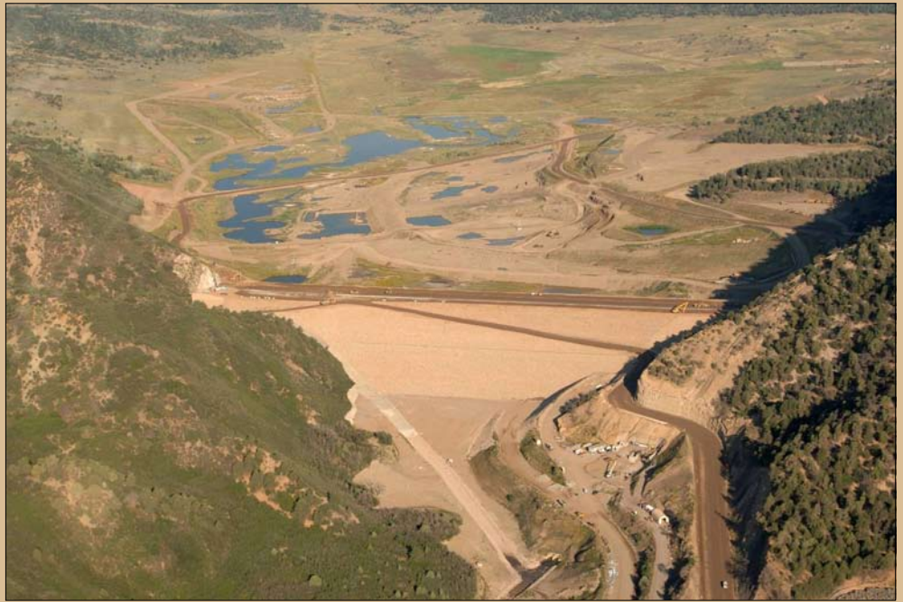
Aerial view of the nearly completed Ridges Basin Dam on Aug. 29, 2007.
