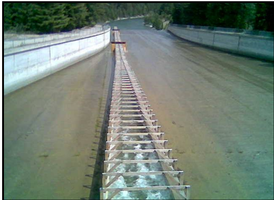
Photo 4. Fish passage flume and PIT tag antennas
