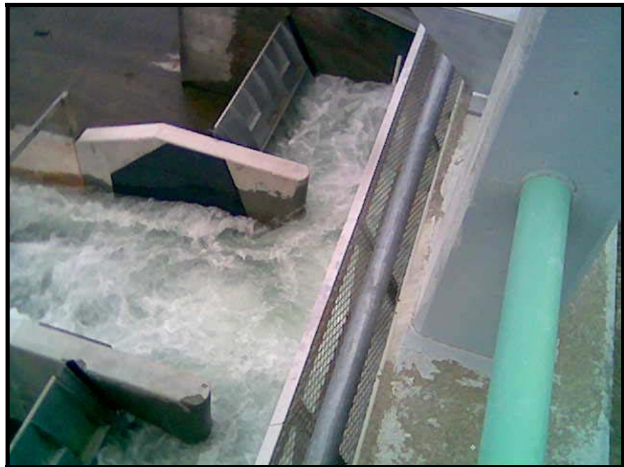
Photo 2. Plunge pool and entrance to flume
