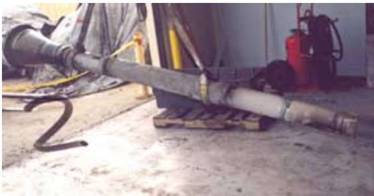
Photo 21: No. 2 engine's fan mid shaft
