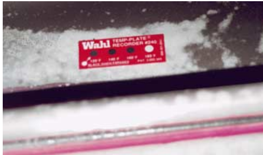
Photo 35: Temp tab over bleed air duct on left side of fuselage showing exposure to 160°F
