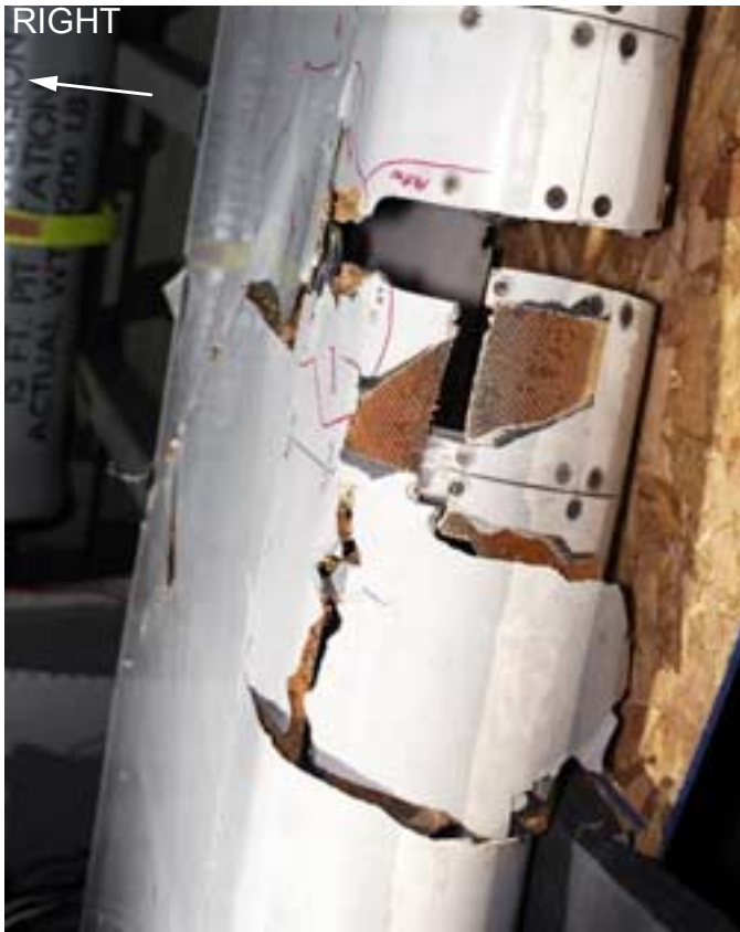
Figure 57. View of the LE fairing at hinge 7.
