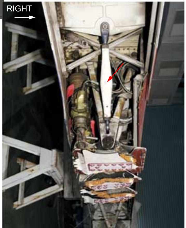
Figure 38. Another view of the hinges 2 to 4 as viewed looking down and forward. The vertical support strut is shown also. An unlabeled arrow indicates damage on the upper side of the support strut.
