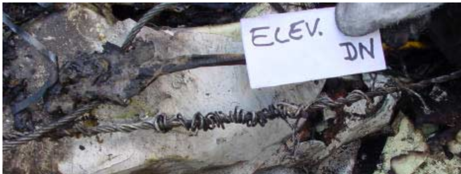
Photograph 11. Elevator down (AND) cable showing spiraled strands.
