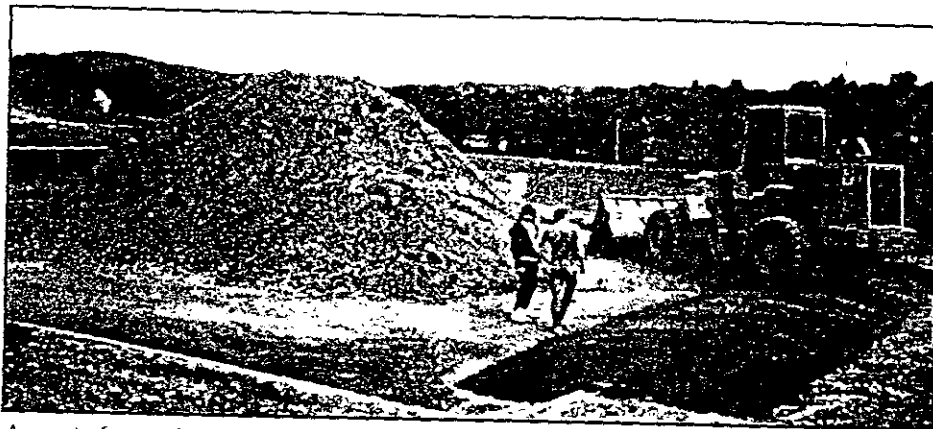
As part of a road construction project in New Jersey, this pile of waste-to-energy ash was left exposed for several months and carefully monitored. There was no hazardous leachate or other environmental problem.
