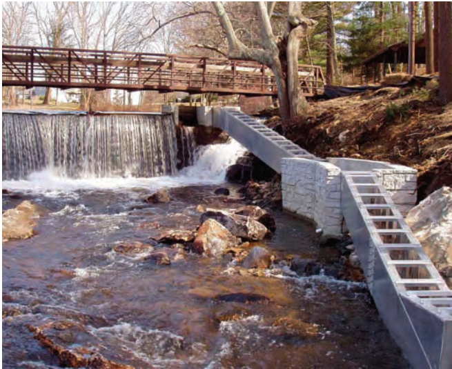
Fish Ladder at Jordan Mill Pond, Waterford, Connecticut, created using settlement funds from the RTC 380 oil spill.
