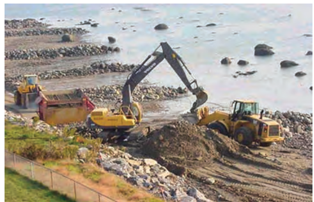
Lordship Point, a peninsula at the mouth of the Housatonic River estuary, had a firing range for a gun club where lead shot was used and entered the environment from the 1920s to 1987. This photo shows the cleanup of contaminated sediments underway.
