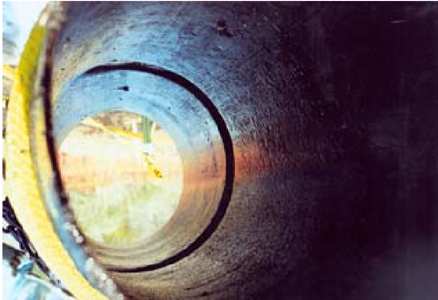
Figure 10. Inside view of the buckle in the removed section of pipe.
