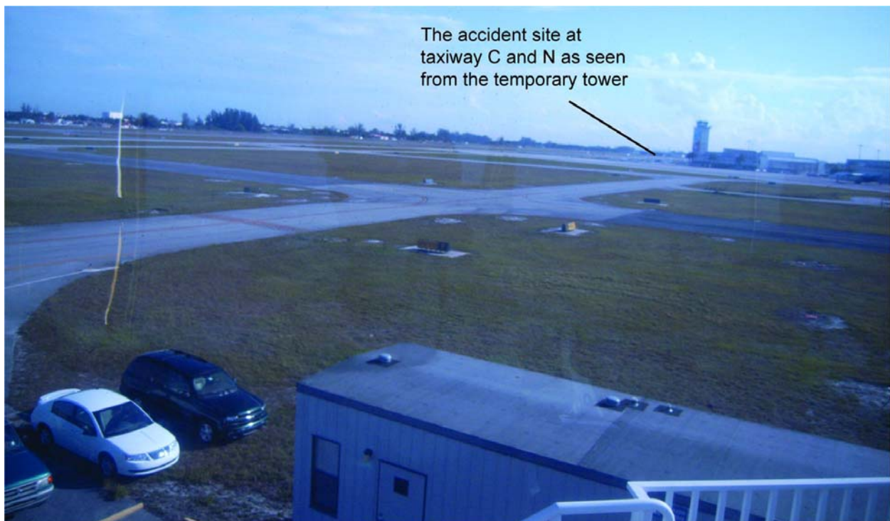
Figure 3. Northwest view of the accident site from inside Opa Locka Airport's temporary air traffic control tower (ATCT). The current location and height of the temporary ATCT prevent controllers from observing aircraft and vehicle movement on the majority of the airport surface and limit some views of aircraft on approach to the airport.
