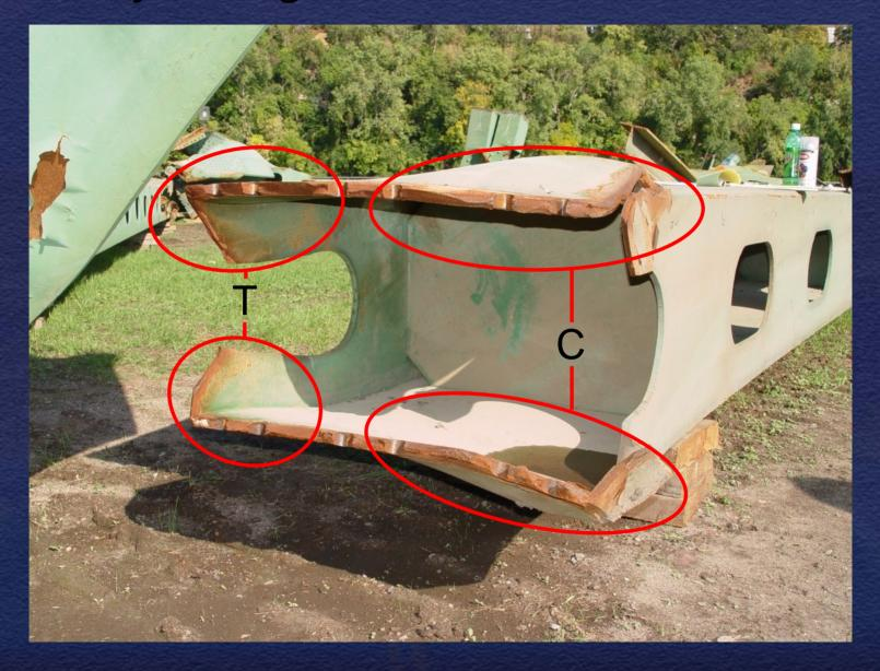
Gusset plates at nodes U10 failed, compression diagonals translated to the west, and remaining portions of nodes U10 were pulled down and through diagonals
