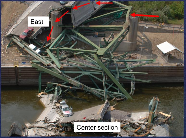
5. Gusset plates at node U10' failed, and additional secondary failures in this portion of the truss completely separated the center section of the center span from remainder of deck truss
