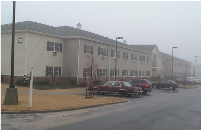
Figure 5 Representative Long Island Multi-Family Building
