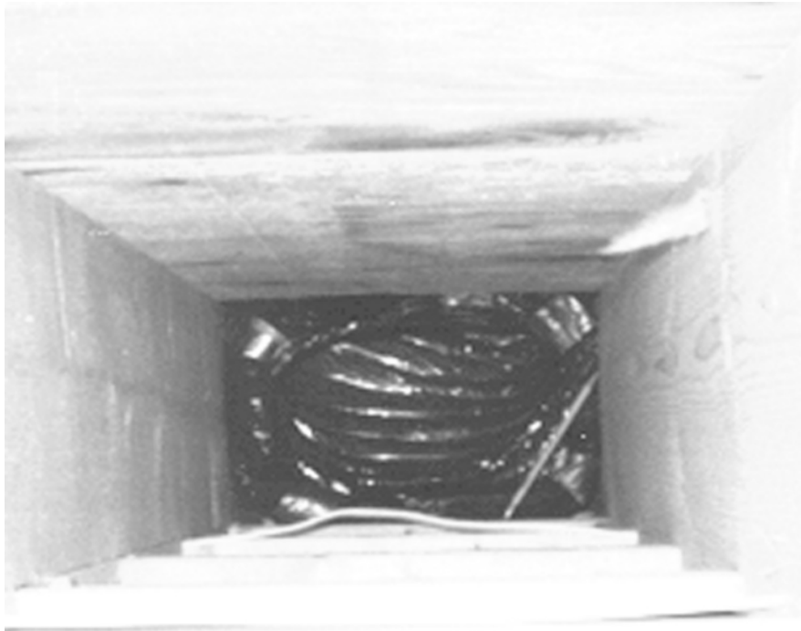
Figure 5-5 Round Duct in a Rectangular Space
