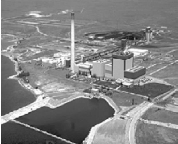
Additional generation is being added at the Platte River Power Authority's Rawhide Energy Station. Natural gas combustion turbines will be ready to meet growing summer peaking needs in 2002.
