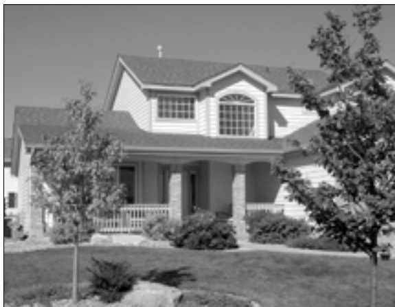
Rooms on the upper levels of two-story homes were often reported to be cool in winter and/or too warm in summer (even in air-conditioned homes).
