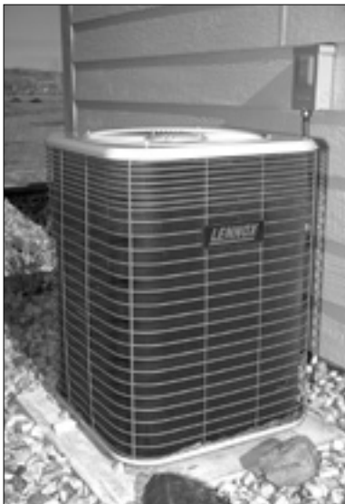
About half the study homes had central air conditioning. The compressor and condenser were located in an outdoor unit like this, with the expansion valve and evaporator coil located in the supply plenum at the furnace.
