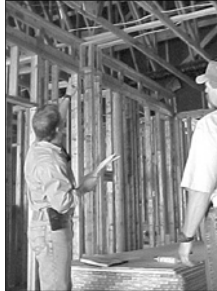
City building inspectors spot-checked compliance with energy code requirements.
