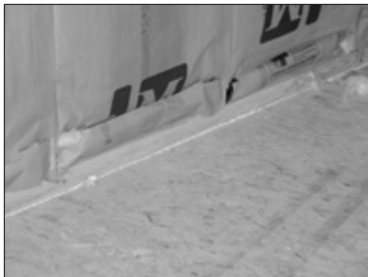
Sealing the baseplate-to-subfloor joint cut off a significant air leakage path.
