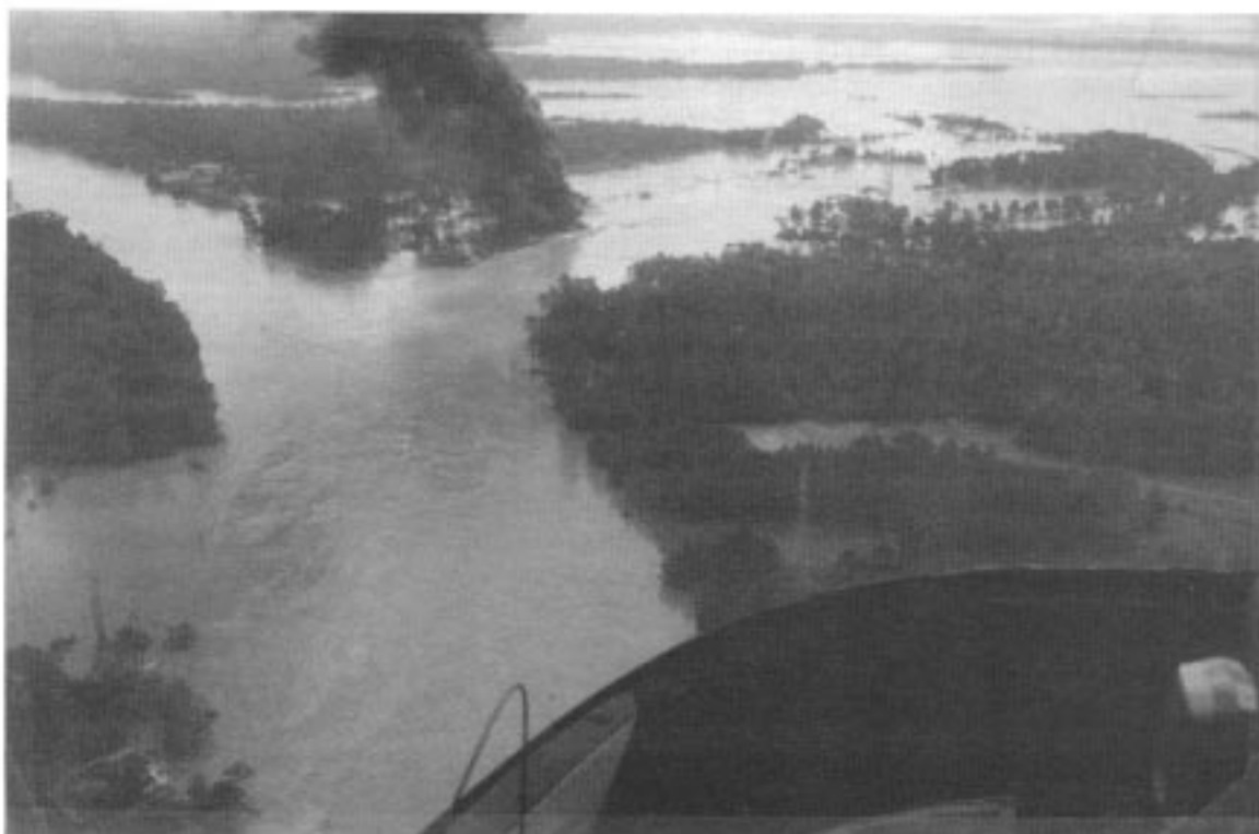
Figure 5 – Fire at ruptured pipeline on east bank of new channel
