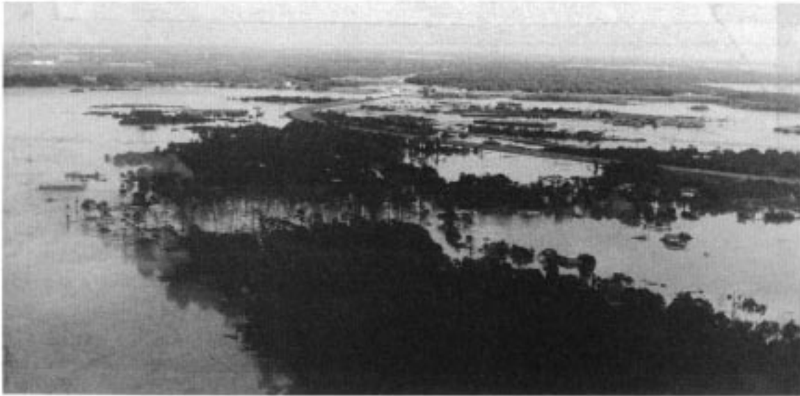
Figure 2 – View of the flooded community
